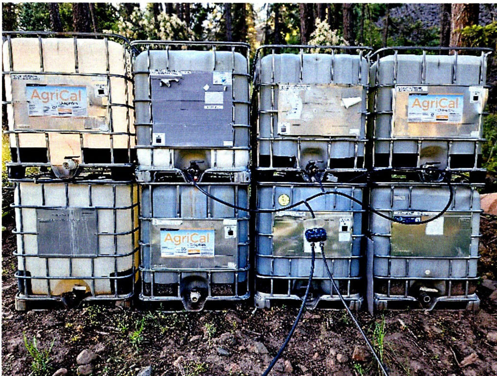
Figure 2. Photo of storage tanks (8 x 275 Gallons) and manifold with timers for ½ inch poly pipe to driplines at trees and attached. Poly lines for the garden or home are connected directly to manifold as needed. Hose hooked up directly for sprinkler to water grounds.
