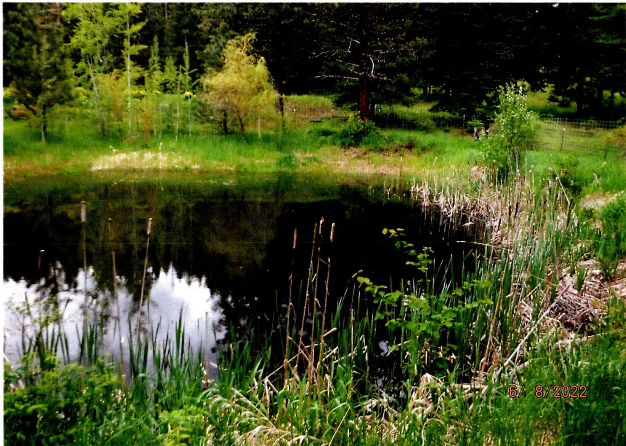
POD – LOWER PONDING EARTHEN DAM
