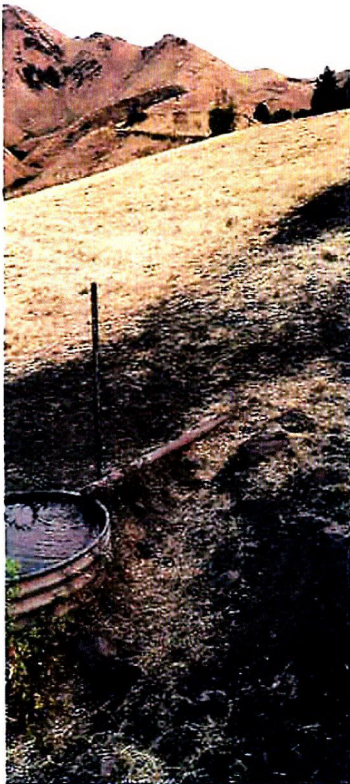
pipe inserted horizontally into spring, draining into stock tank, above, below left
