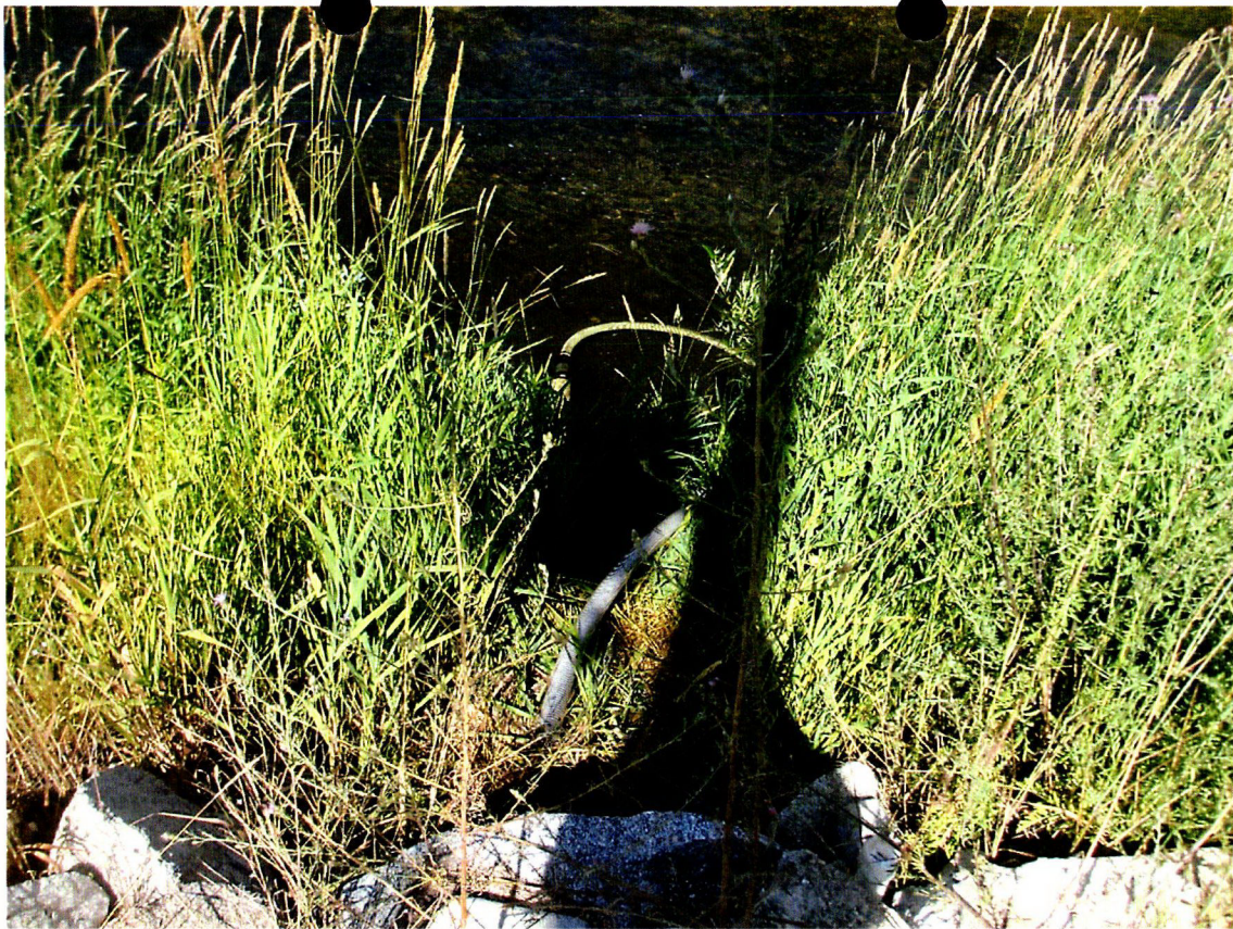
Point of Diversion – inlet hose in Middle Fork of the Payette River
