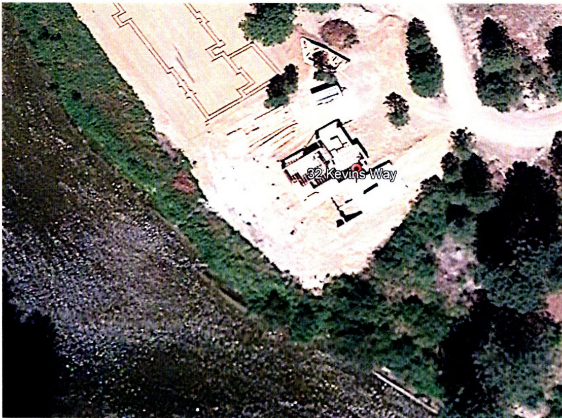
Figure 1- Google Earth, 2022 aerial imagery of the POU. Construction is still incomplete.
