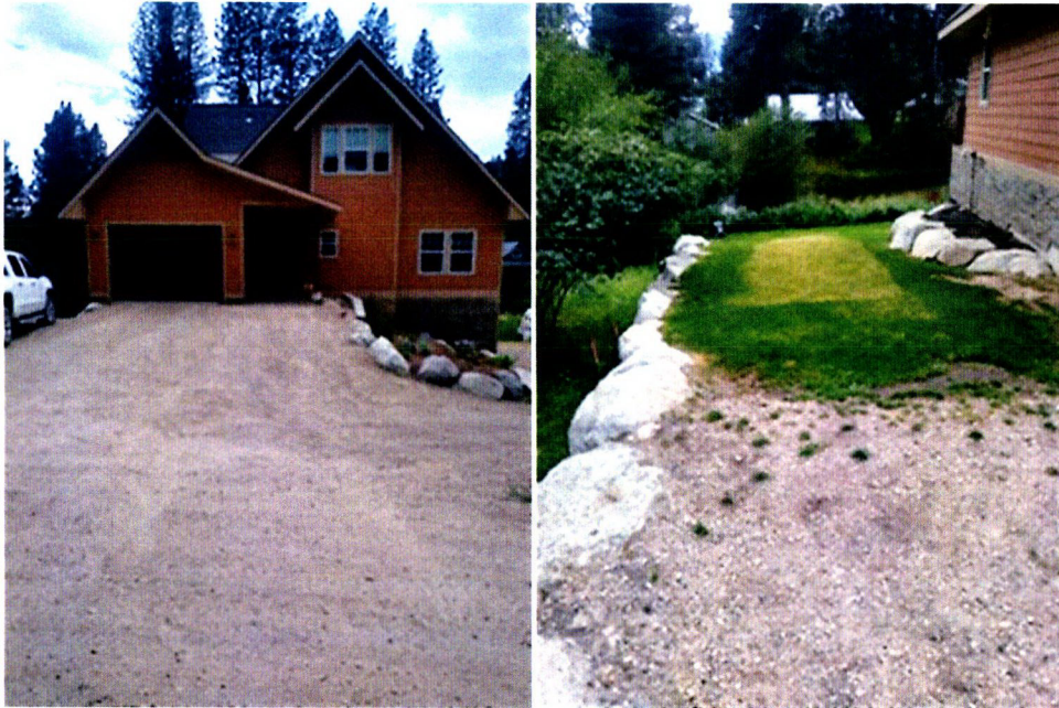
Photos 1 & 2- Facing the SW center and left of the house (SE side of home).
