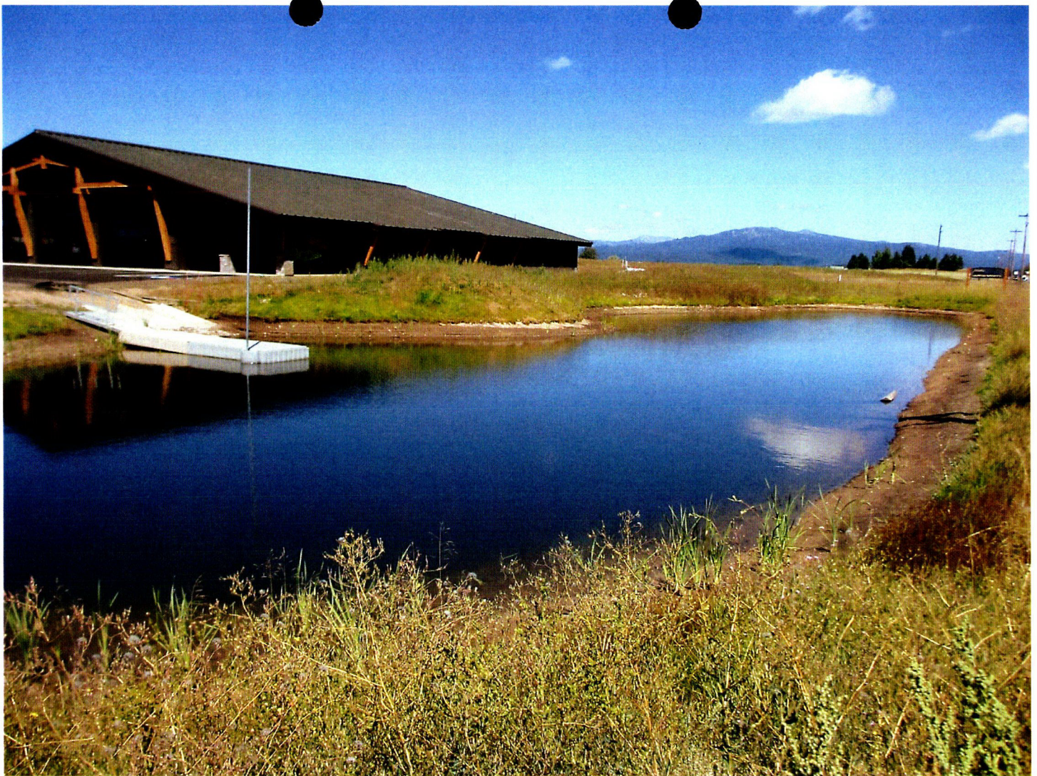
Point of Diversion and Place of Use (excavated pond intercepting ground water).
