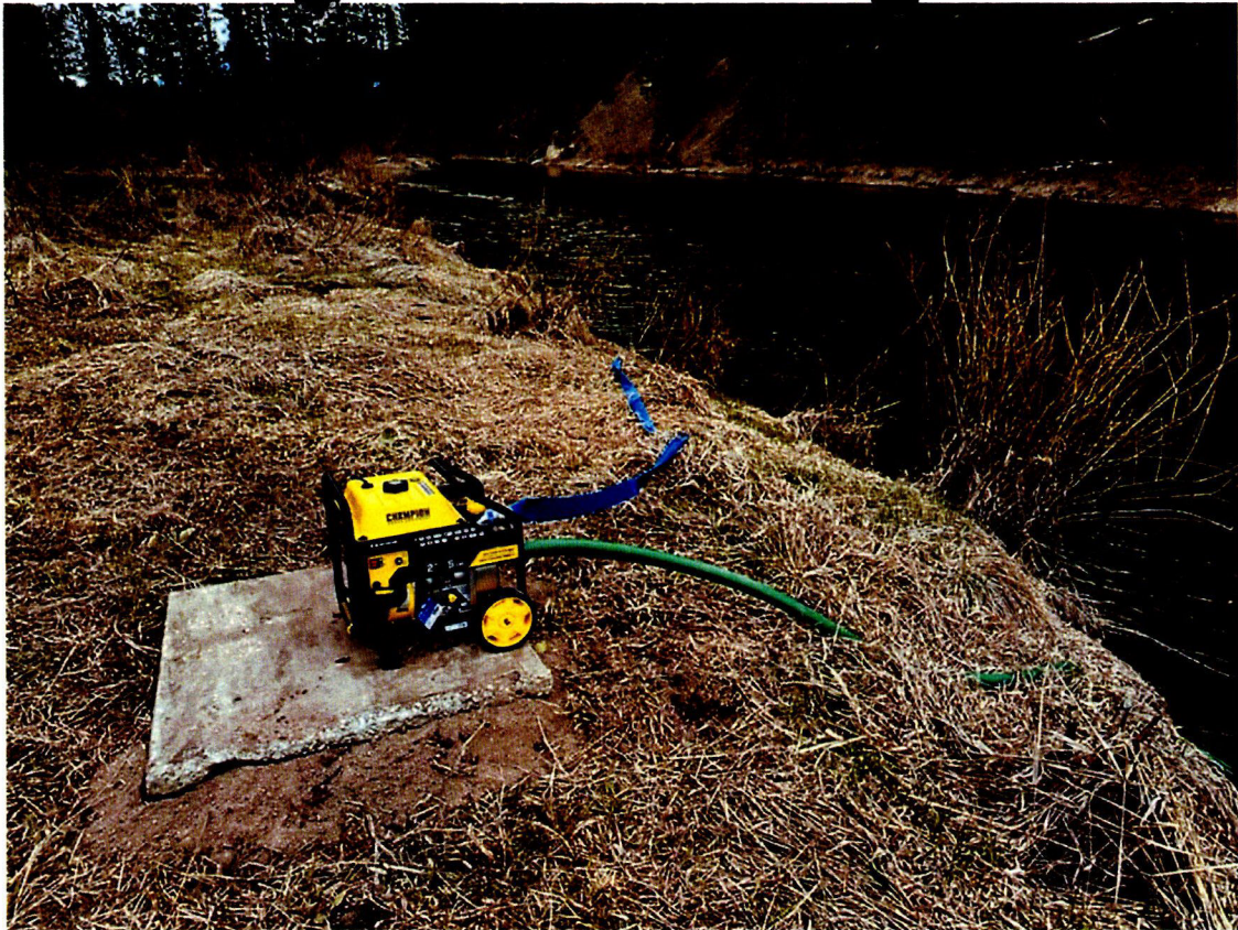
Point of Diversion - Portable gas pump in river
