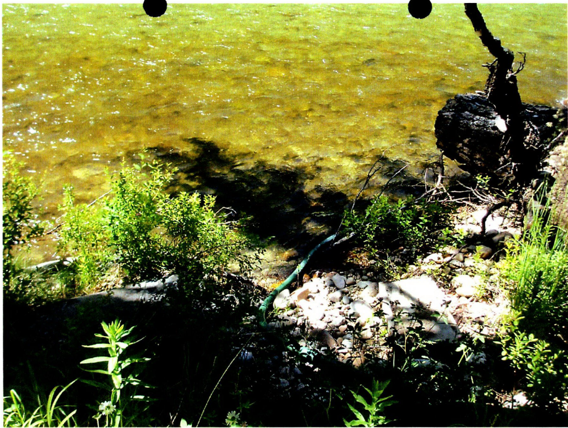
Point of Diversion – Suction hose in river
