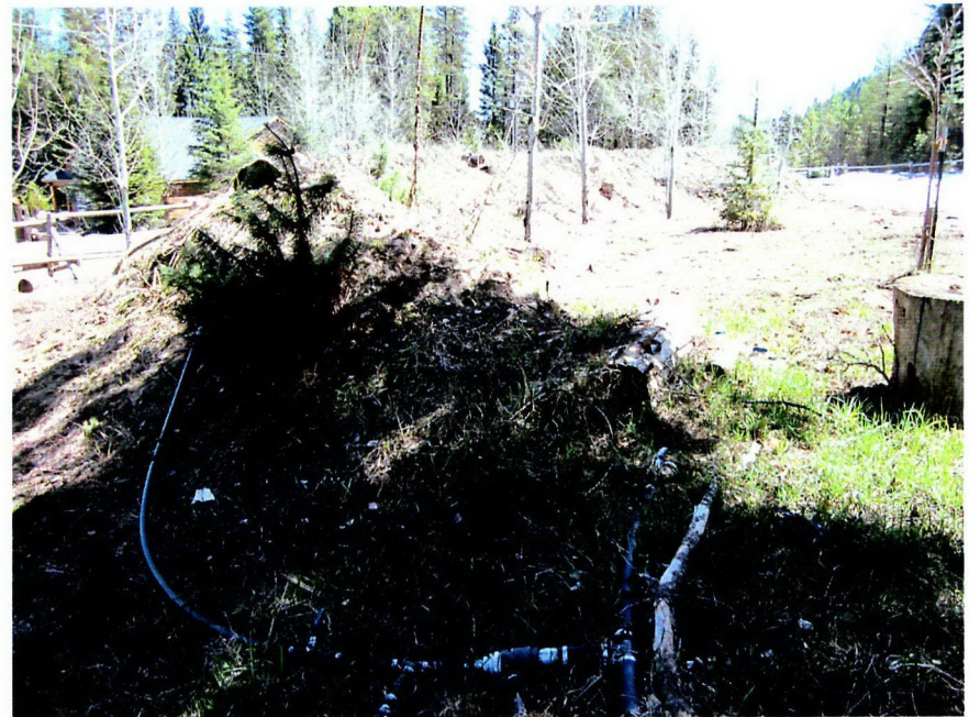
POU east of house (irrigation pipes)
