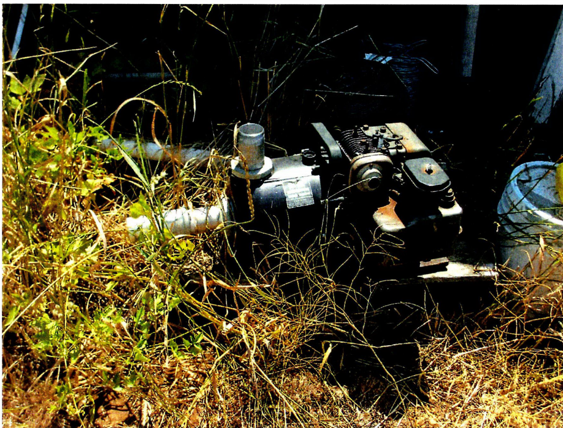
Pump used to divert water
