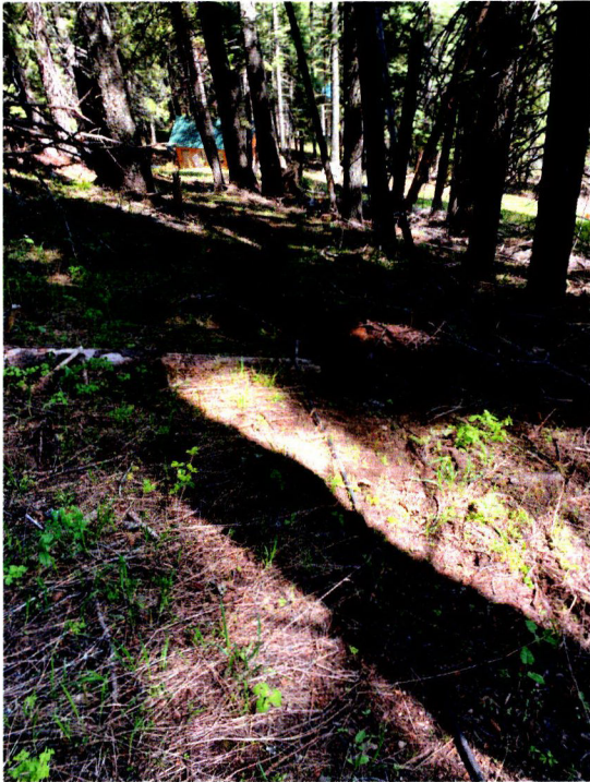
Water line going to four containers
