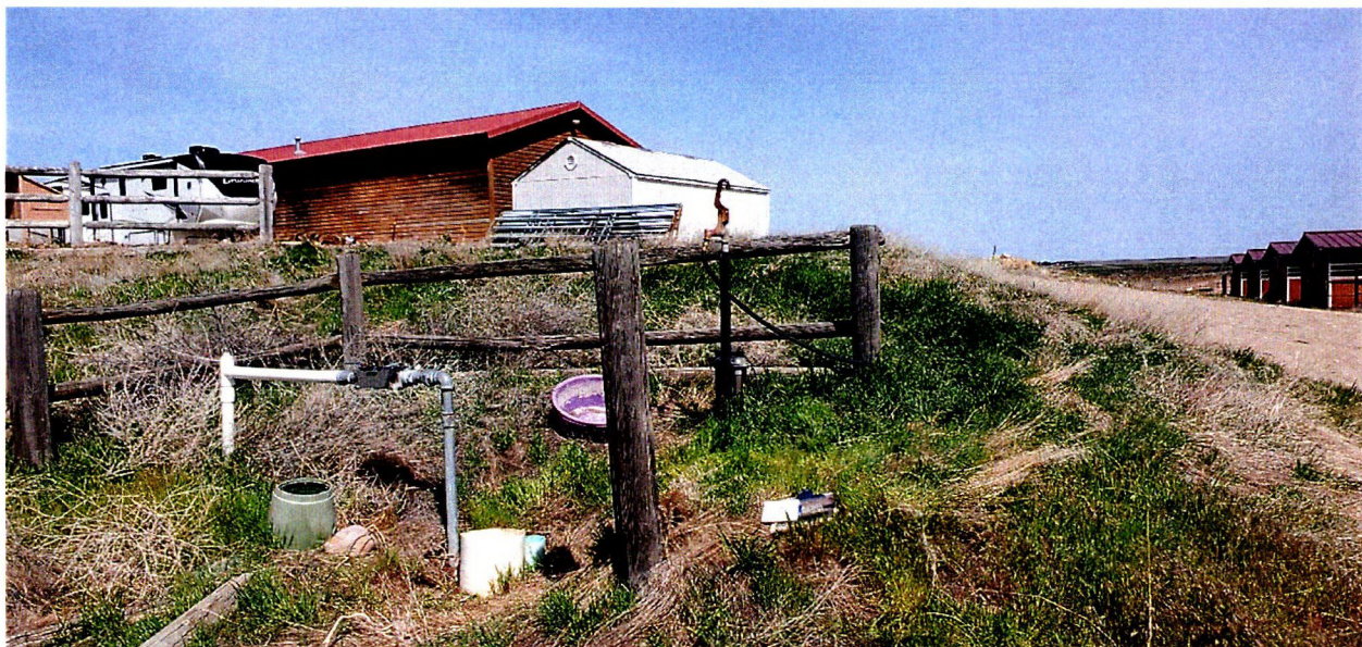
Figure 2: Domestic/stockwater well (just behind hydrant)
