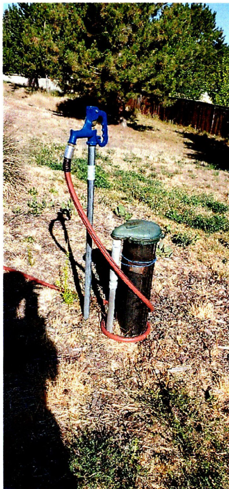
Figure 6: Well head
