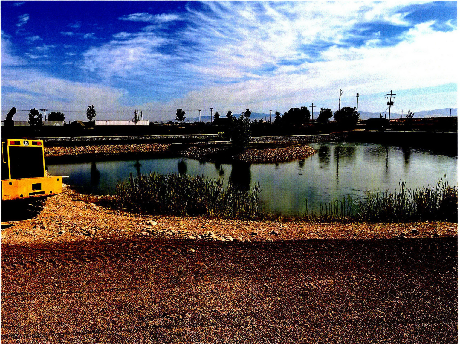
Fig. 5 – W side facing toward center island of pond.
