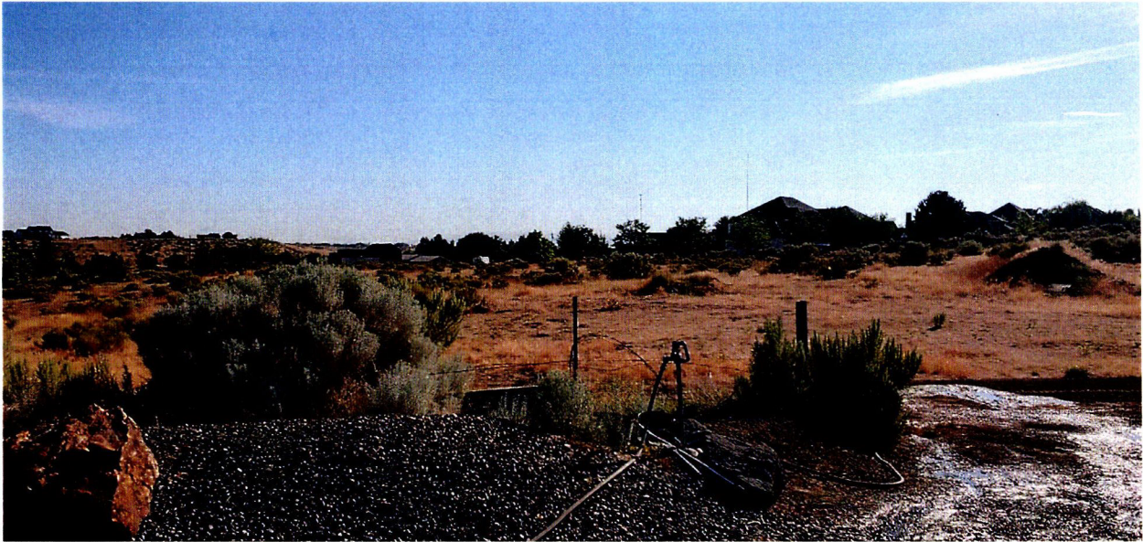
Figure 3: A strategically placed hydrant and a field of sagebrush behind it
