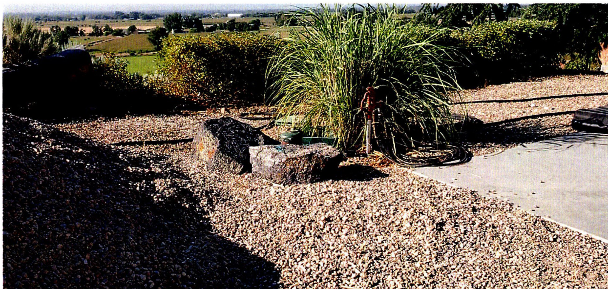
Figure 5: The wellhead, hydrant, and hoses (so many hoses!)
