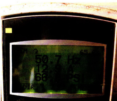
Photos 2, 3, &4: Digital display, pump information, and pressure gage. The readings shown reflect the system operating at higher flows than during typical operational conditions. At these operating conditions and the pump at approximately 12 feet, the theoretical flow rate is 0.18 cfs (83 gpm), which is reasonable. The water right permit allows a diversion rate of 0.12 cfs
