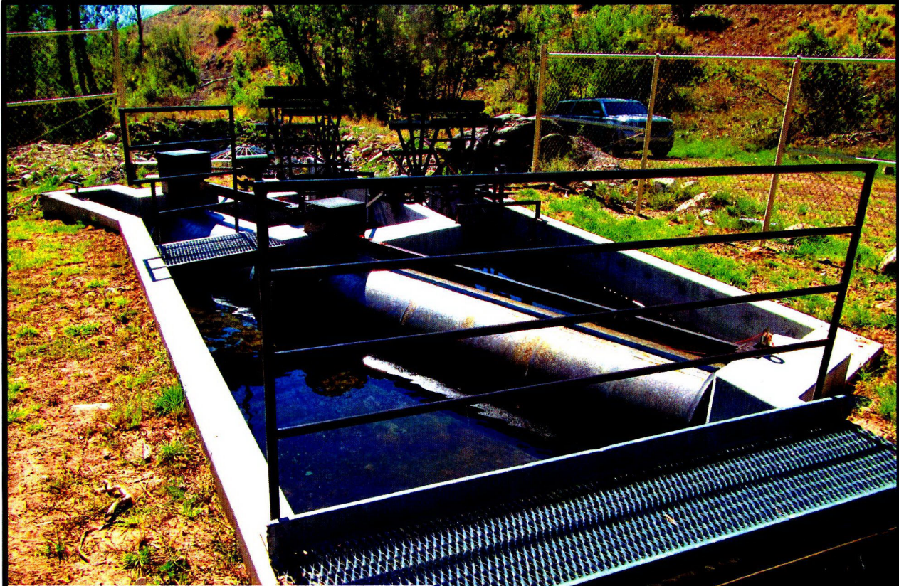
Fish screen with bypass pipe flow (.80 cfs) returning to Pratt Creek
