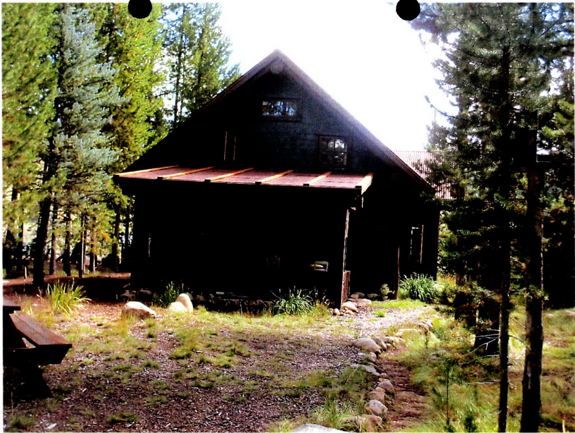
Domestic POU – Typical home in the subdivision
