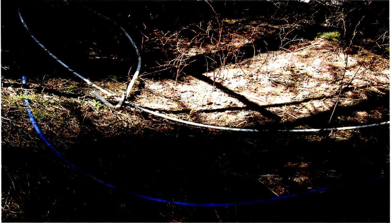
Above: Additional pipes for Irrigation
