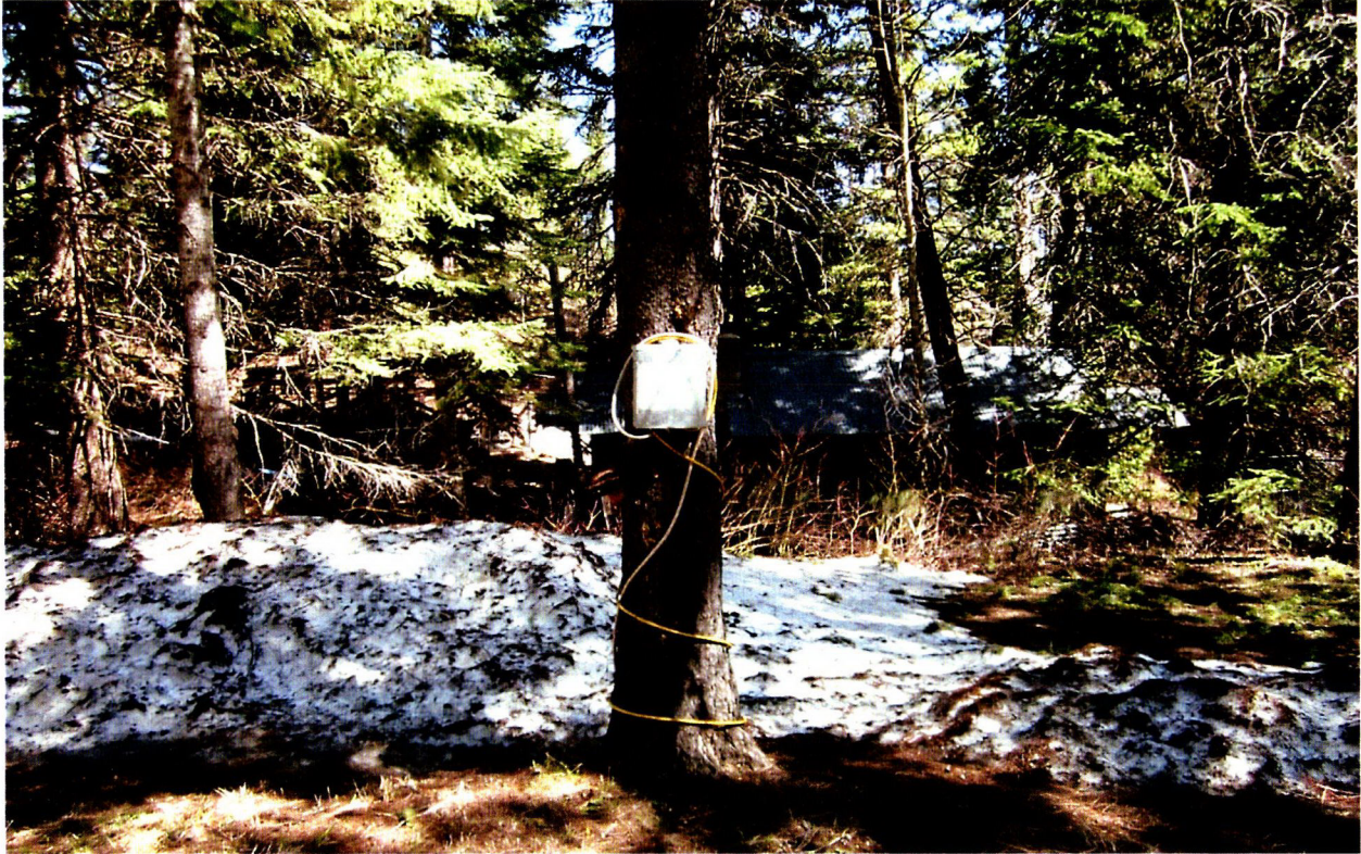
Above: Lockable controlling works, and Irrigation
