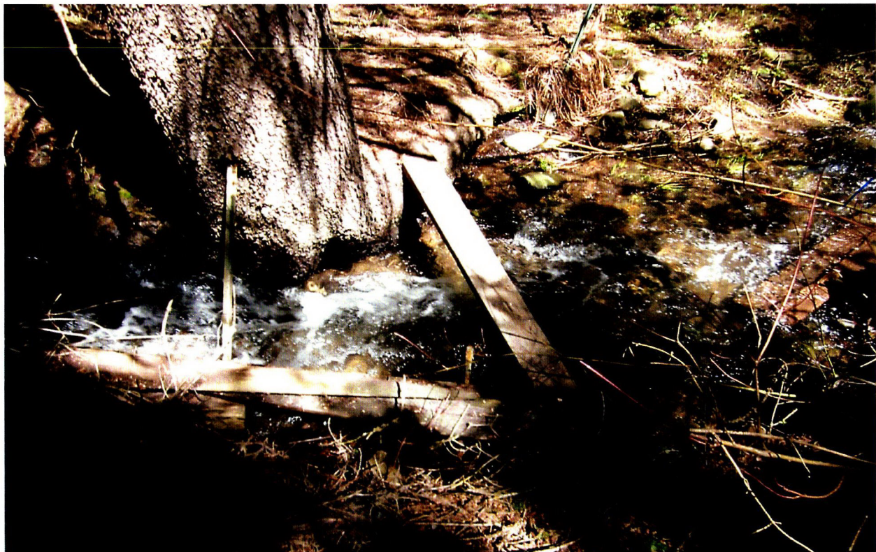
Below: Point of Diversion for pump from unnamed stream
