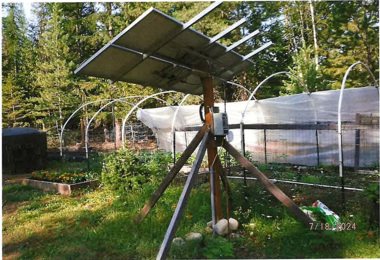
RSP PUMP CONTROLLER AND SOLAR PANEL CONFIGURATION
