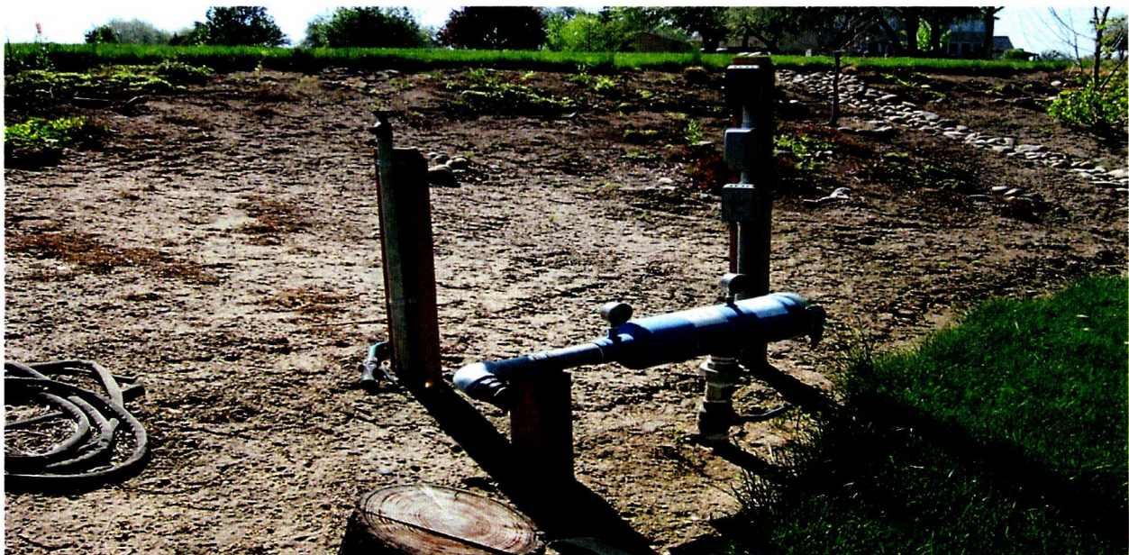
Connection of 2" hose from pump to pressurize system
