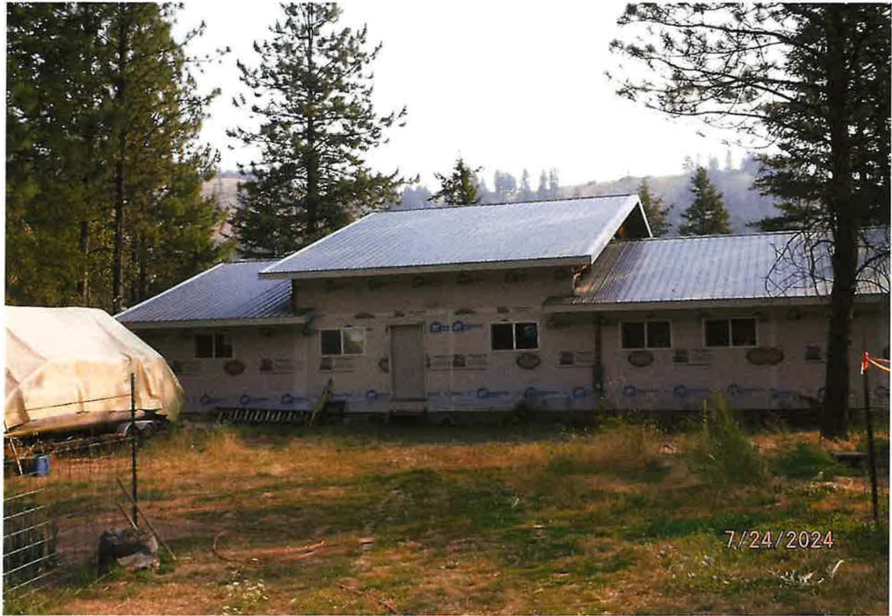
DOMESTIC POU – 4 TH HOME WITH LAWN AND GARDEN WATERING. PARCEL RP36N03E181645
