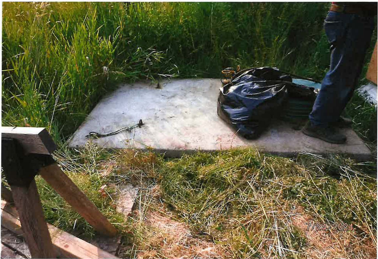
OVERFLOW WATER FROM 2,400 GALLON RESERVOIR FILLS SECOND 1,200 GALLON VAULTED RESERVOIR
