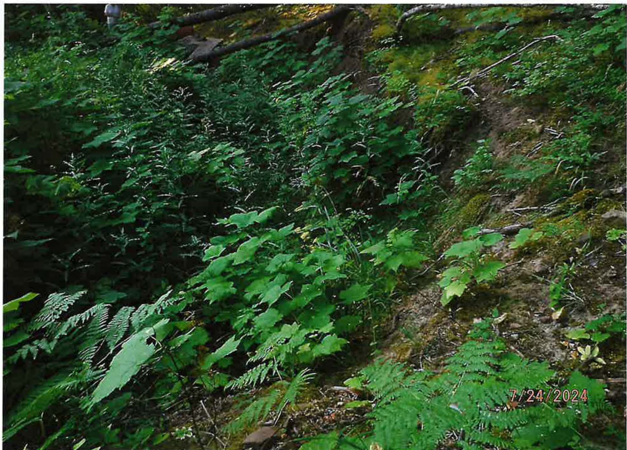
POD – SPRING SOURCE EXCAVATED TO 12 FT BEFORE DRAIN TILES WERE INSTALLED, COVERED WITH FILTER FABRIC & ROCK PRIOR TO EARTHEN OVERLAY TO PROTECT SPRING FLOWS FROM CONTAMINATION
