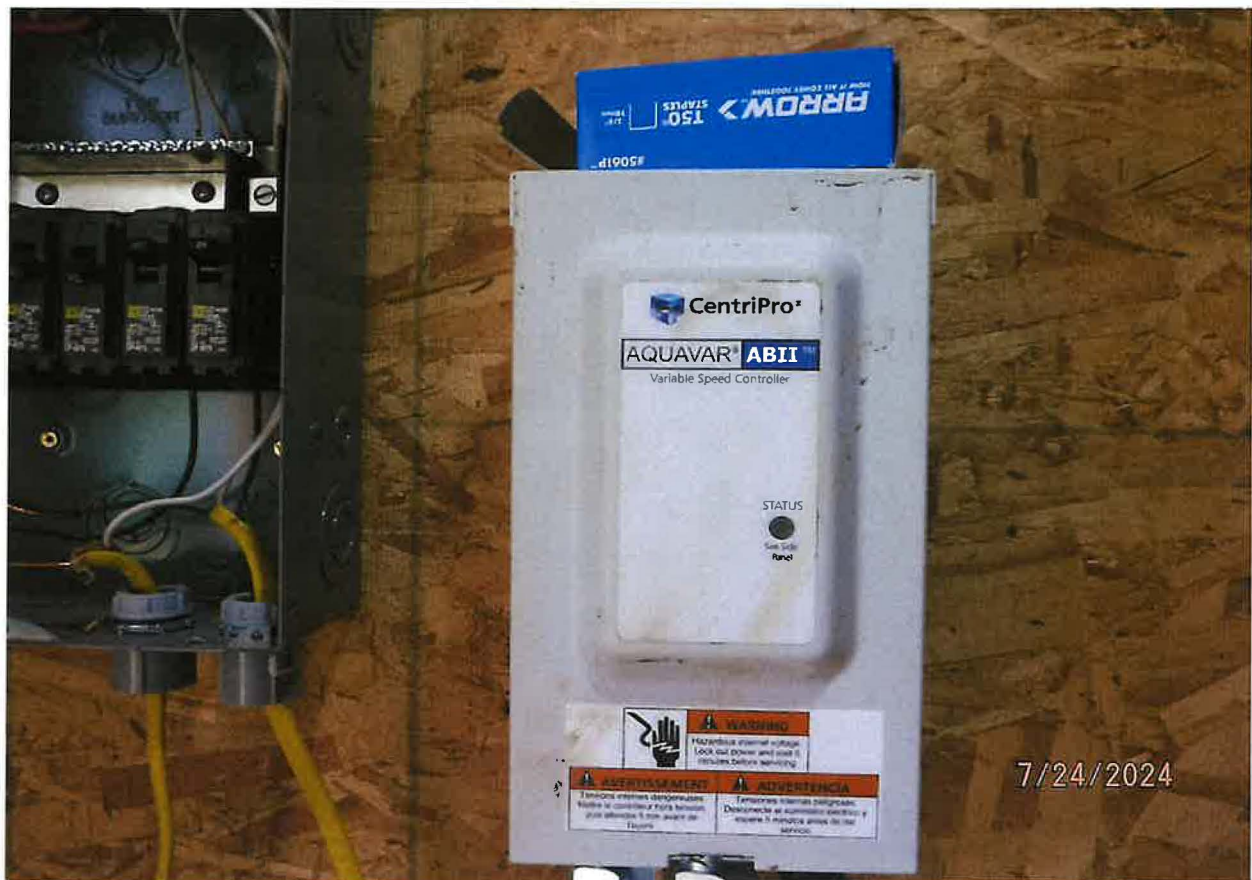
CENTRIPRO AQUAVAR PUMP MOTOR CONTROLLER
