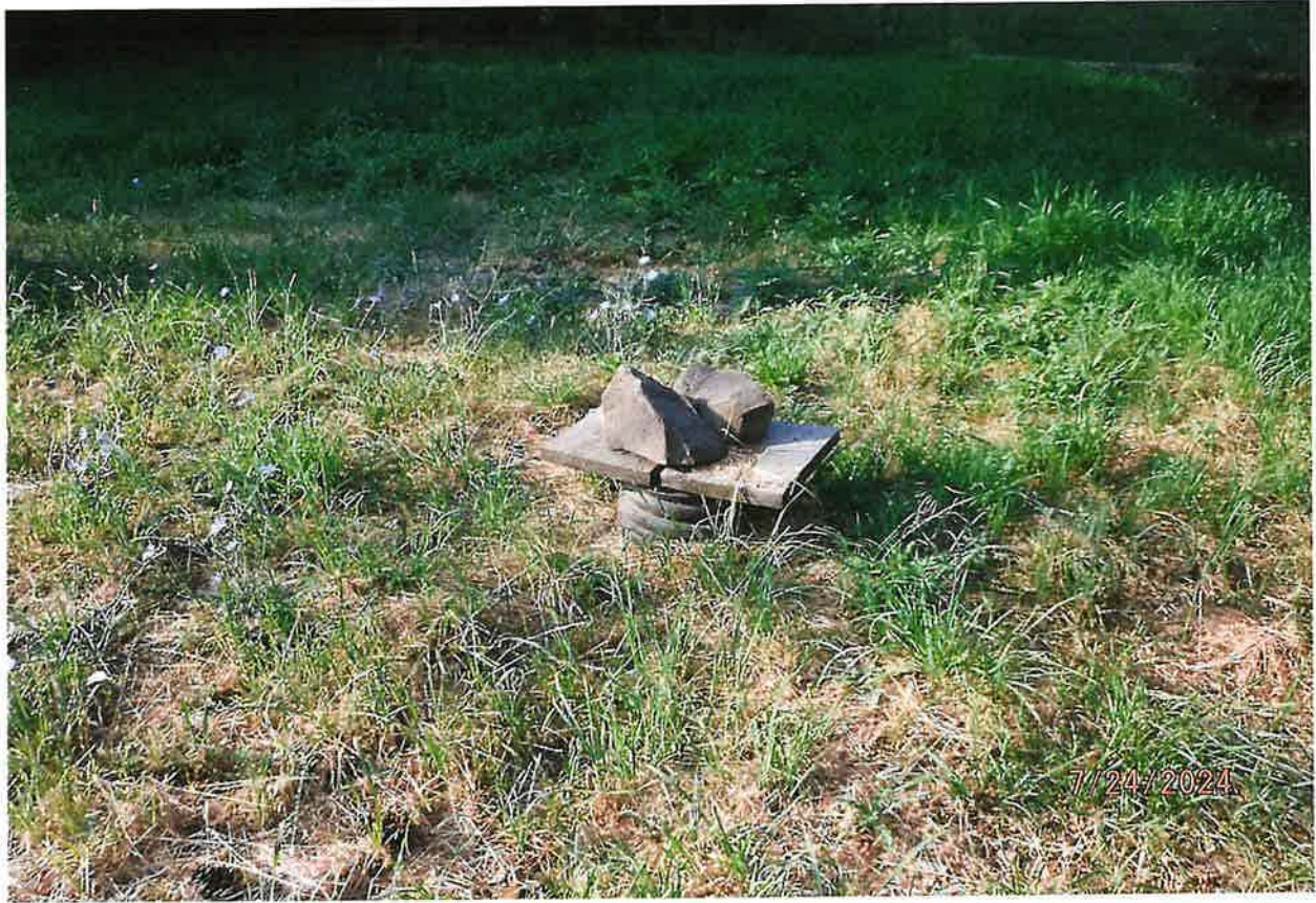
MANUAL SHUTOFF VALVE FOR 3 RD HOME SERVICE CONNECTED TO WATER SYSTEM
