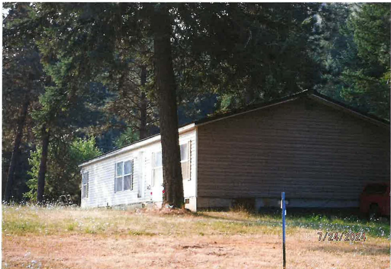
DOMESTIC POU – 3 RD HOME WITH LAWN AND GARDEN WATERING. PARCEL RP36N03E188410
