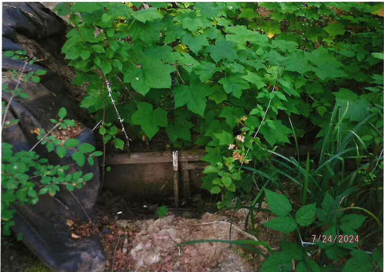
CONCRETE DAM 7 FT TALL IN SPRING EXCAVATION CONTAINS SPRING FLOW ADDING HEAD PRESSURE TO GRAVITY FLOW PIPE FROM DRAIN TILES
