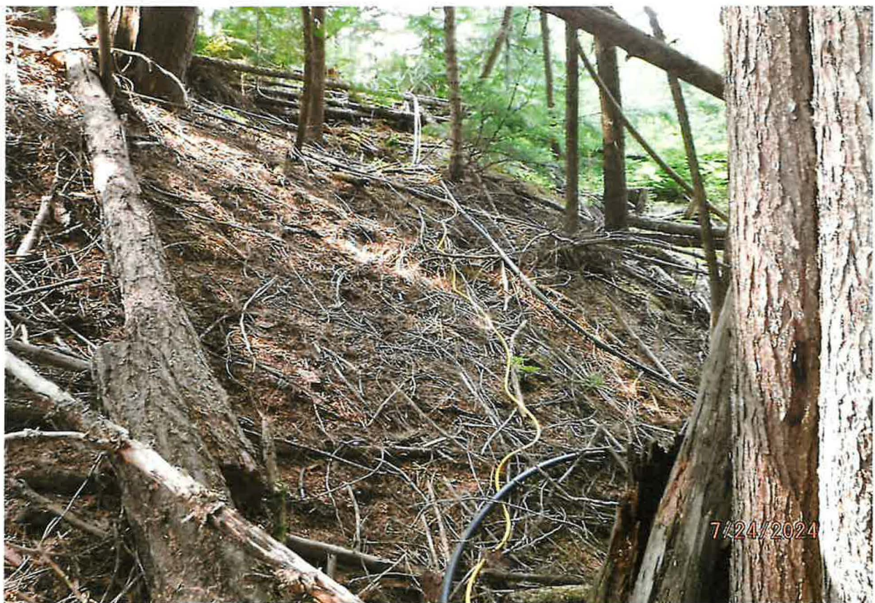
POLY-PIPELINE ROUTES UP-SLOPE TO THE POU FROM STREAM POD
