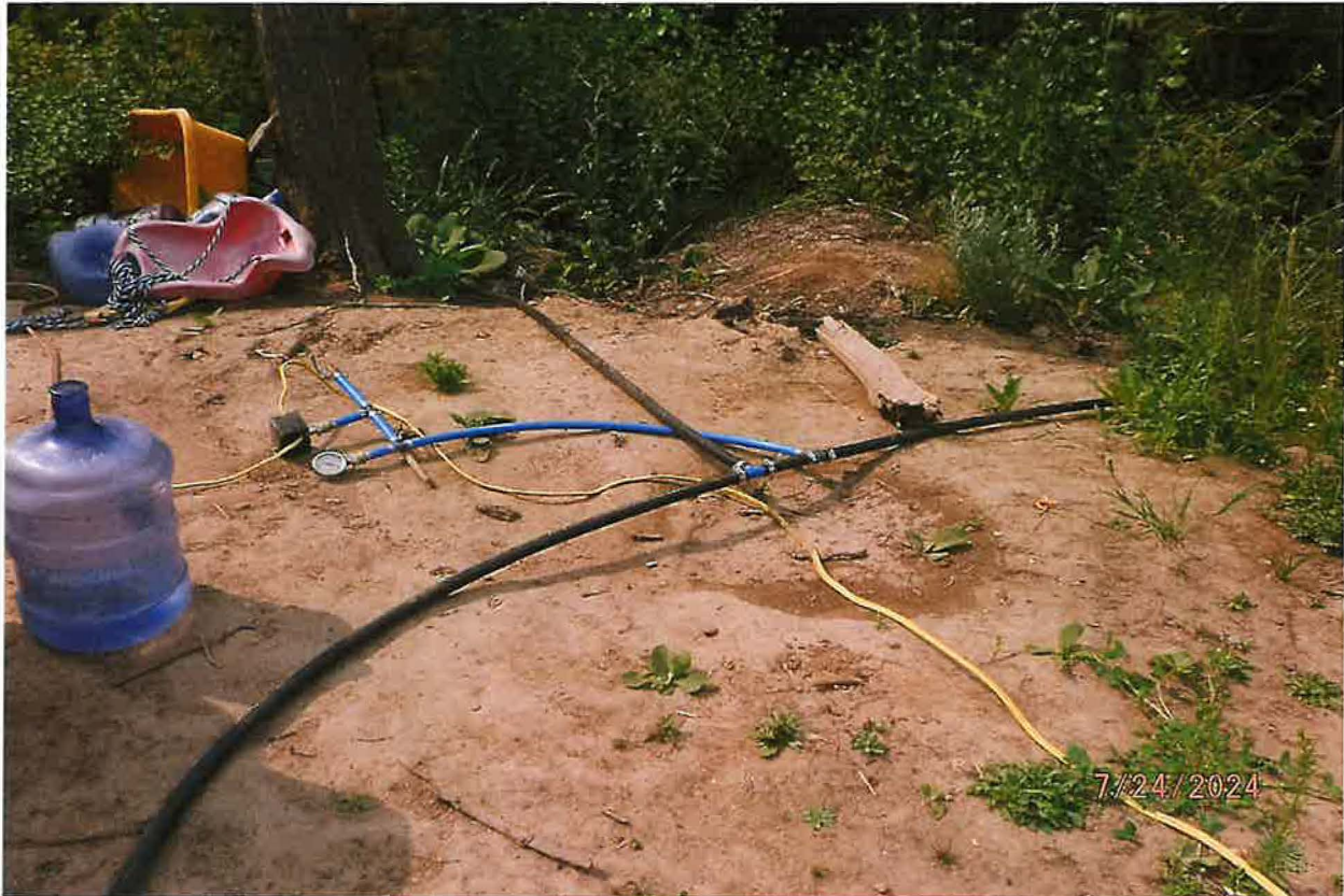
GENERATOR OPERATED 1 HP PUMP IN CISTERN DELIVERS STREAM WATER TO POU
