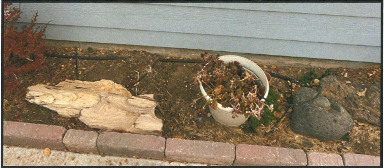
Photo 14- Driplines for watering the landscaped beds around the home (zone 2).
