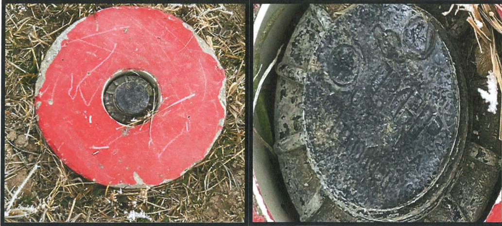
Photos 11- (above) -Hunter PGP Ultra sprinkler heads poured into concrete bases. Sprinkler heads are positioned along the fence lines of zones 3 & 4.
