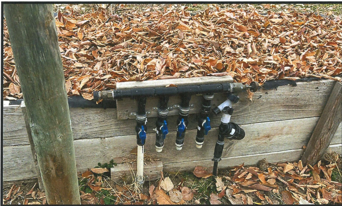
Photo 5 (above) - South of the driveway facing west. The garden beds with drip system. Photo 6 (below) - The manifold for the drip system on the south side of the property and hose bibs for hoses and sprinklers.
