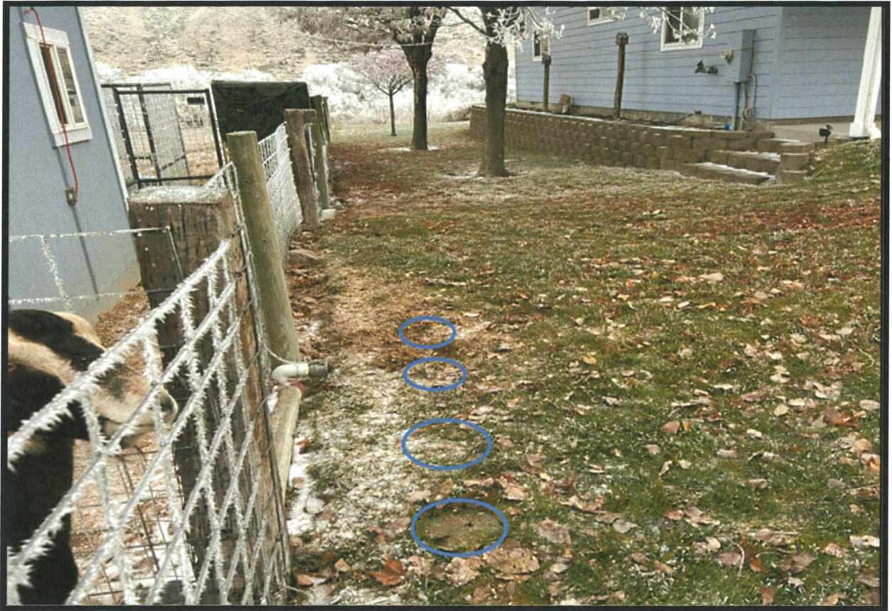
Photo 3 (above) – The four blue ovals in the image outline the overgrown control valves. Photo 4 (below) - Two blue ovals outline control valves 3 &4.
