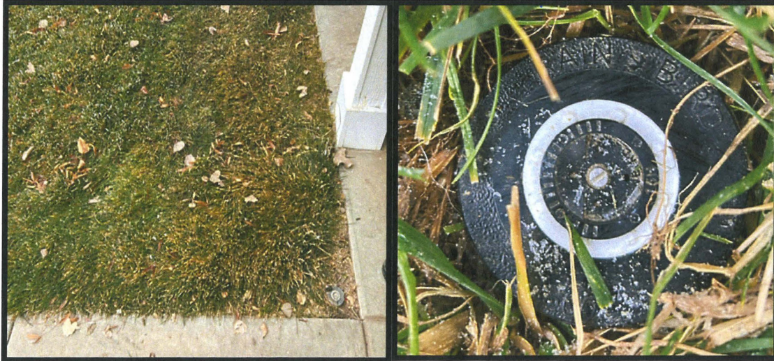
Photos 12 & 13 (above)– Rain Bird 1800 SAM Series rotary sprinkler heads as found in zones 1 & 2. Smaller Umbrella Rain Bird 1800 Sprinkler heads are also found in both zones.
