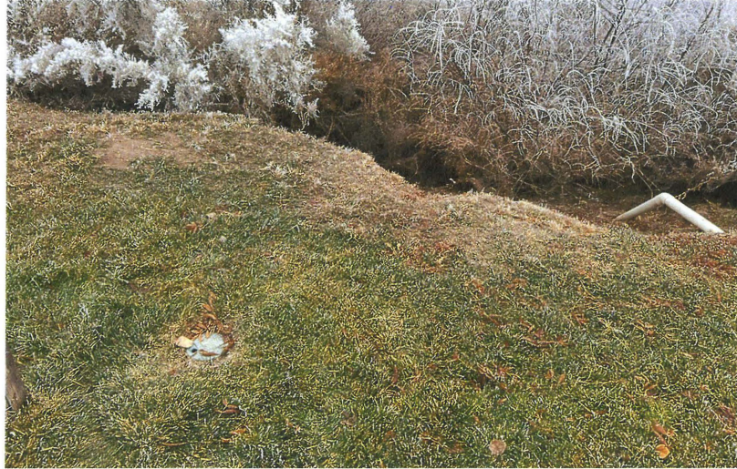
Photo 17- Drain valve and drain pipe north of the northeast corner of the home.
