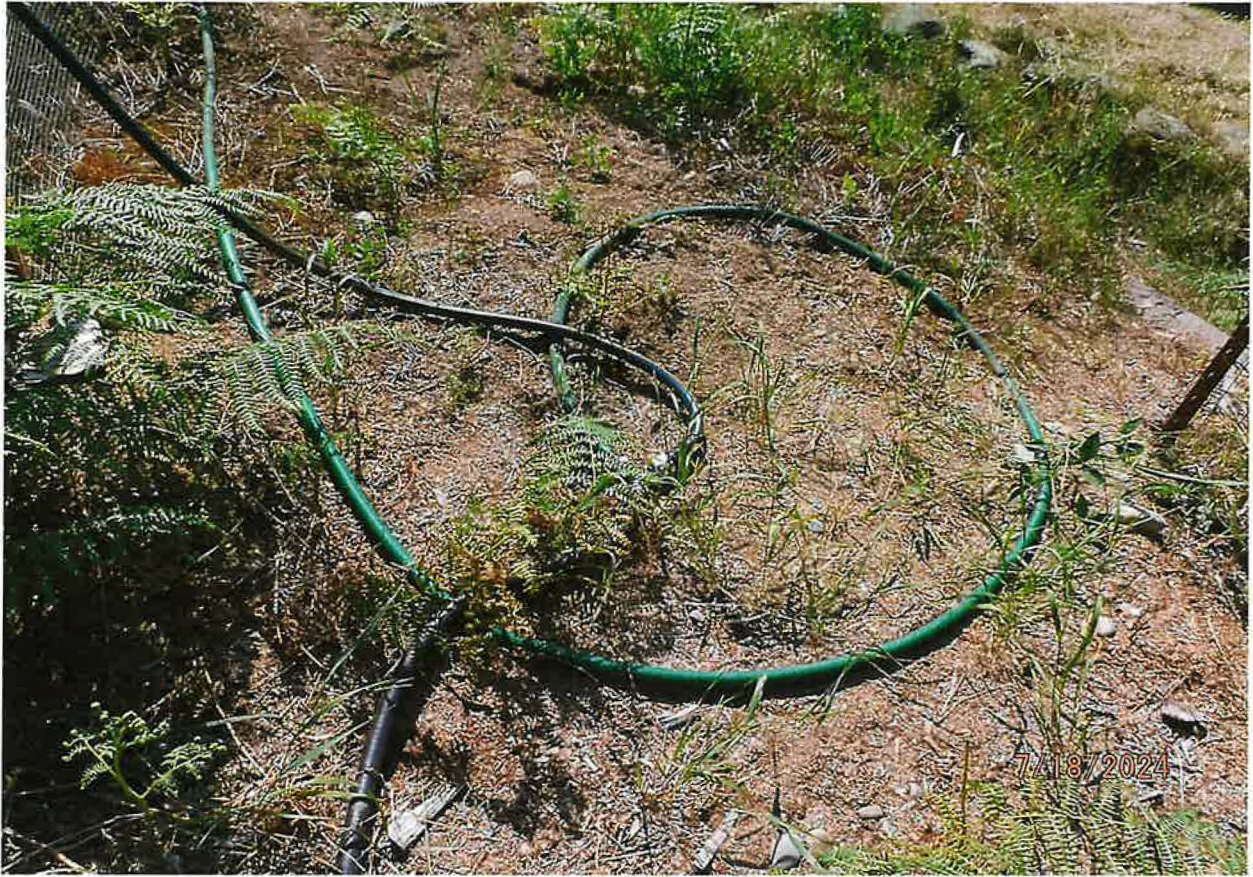
EXAMPLE – HOSE SPLITTERS ROUTING TO DIFFERENT IRRIGATION AREAS WITHIN THE POU
