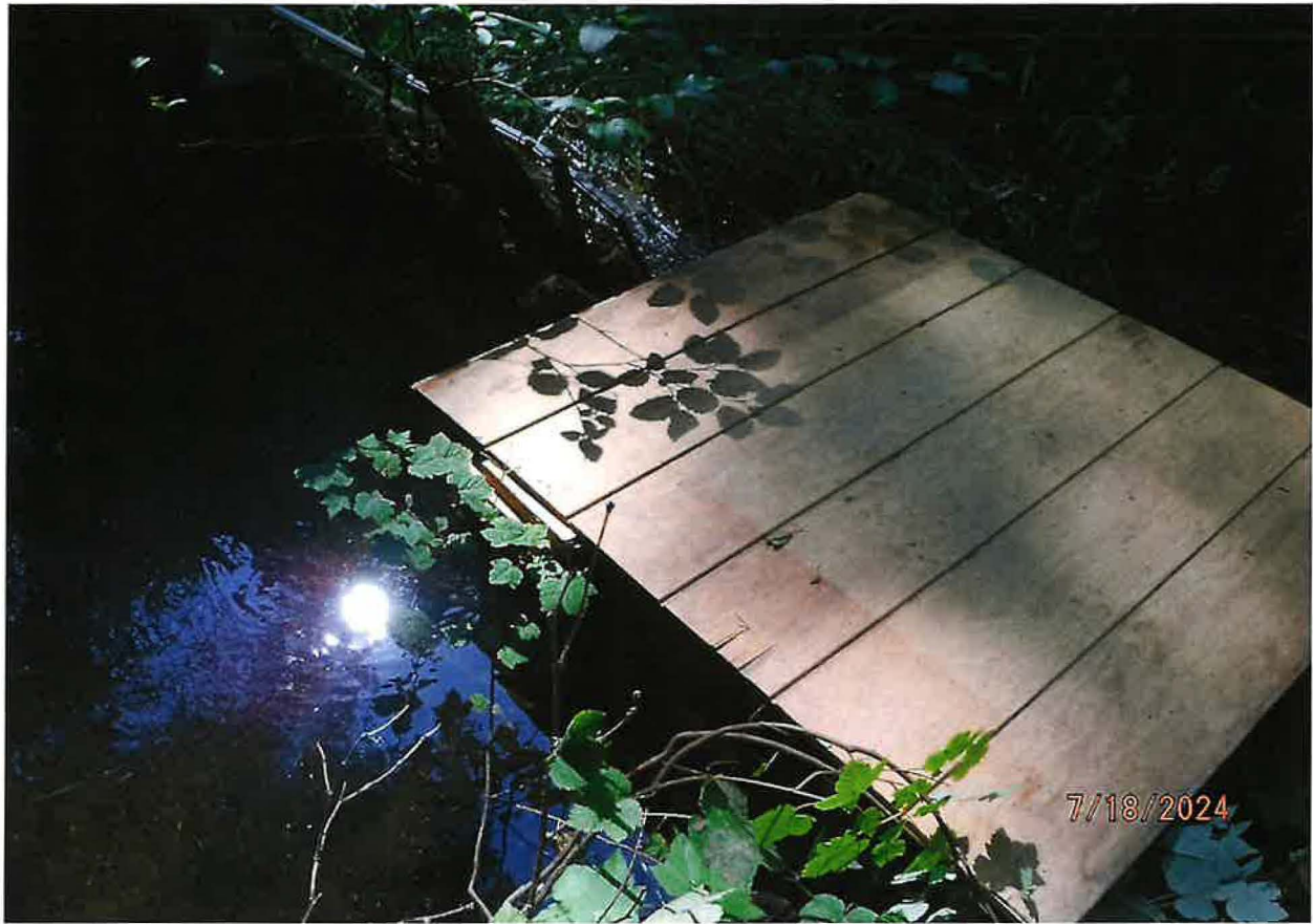
POD – COLLECTION BOX WITH SCREENED PIPELINE FROM CREEK WHICH GRAVITY FLOWS IN CONVEYANCE PIPELINE
