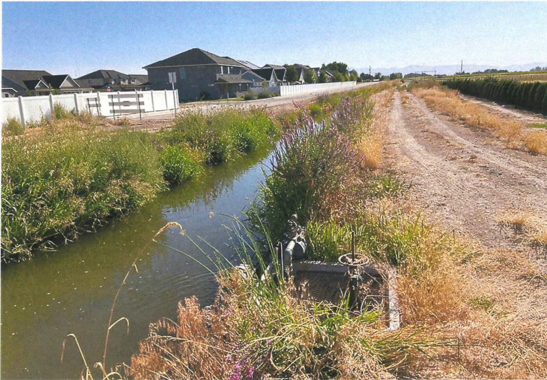
Figure 6 Headgate diversion associated with irrigation from Middleton Mill Irrigation Company. Headgate is located on north end of subdivision.
