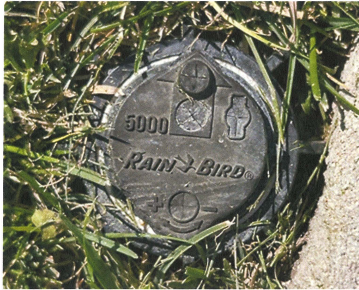
Figure 10 Rain bird 5000 sprinkler head used throughout the subdivision.
