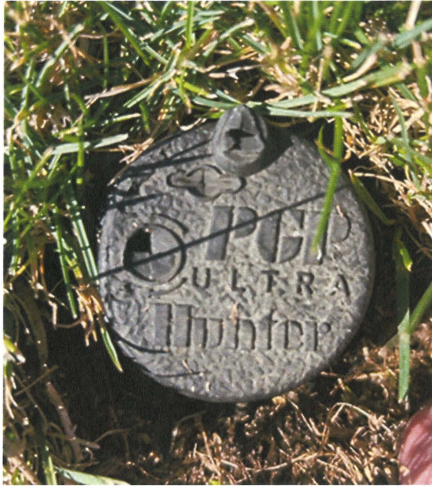
Figure 8 PGP Ultra sprinkler head located throughout the parcel.
