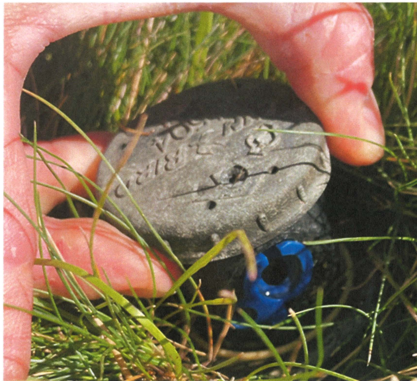
Figure 7 Rain Bird 6504 Nozzle 18 with a flow rate of 19.8 gpm. Sprinkler head found within an irrigated area belonging to the HOA.
