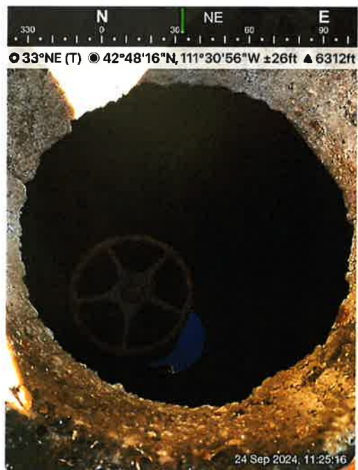
Valve to PVC line inside spring box
