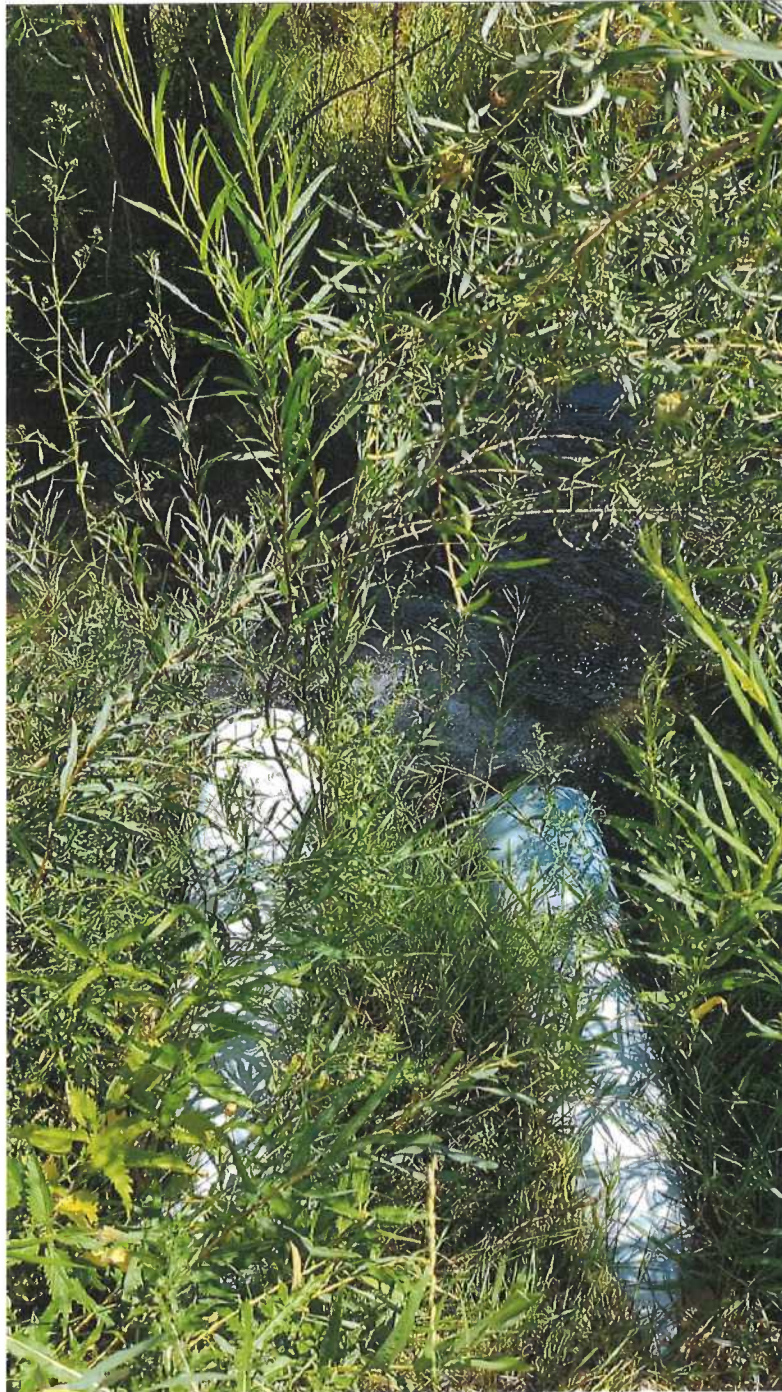
Photo 3: Return flow to Sulphur Creek. Right (southern) 10" pipe is for fish bypass. Left (northern) pipe is overflow from irrigation pipeline.
