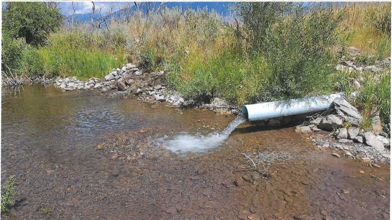
Photos 5 and 6: Return flow to Pahsimeroi River through 10" pipe.
