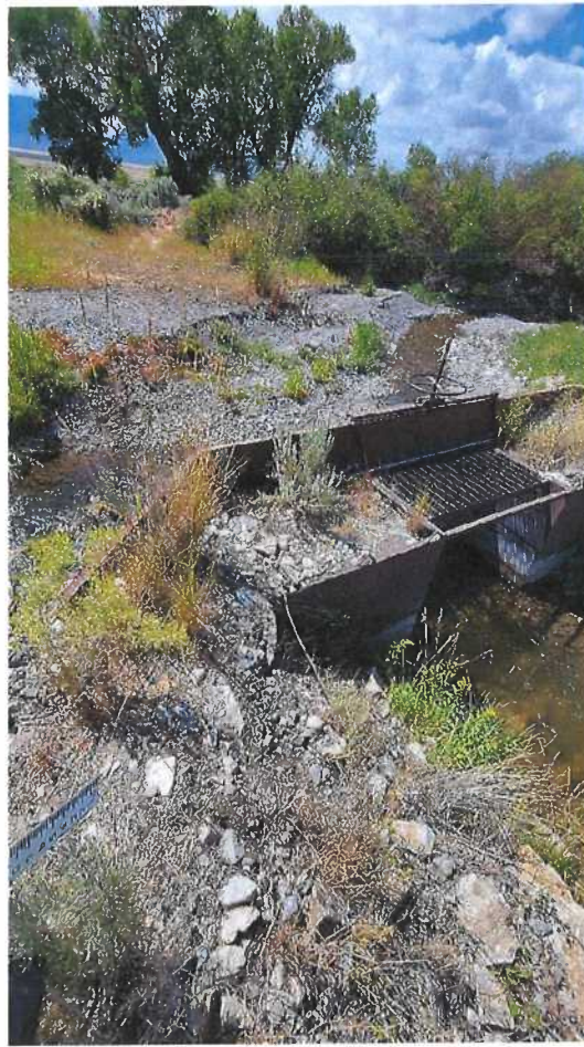
Photos 1 and 2: Diversion and headgate from Pahsimeroi River
