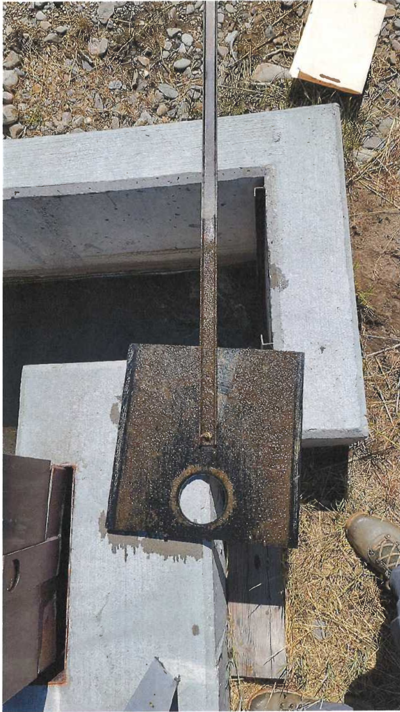
Photo 4: Board with 4" orifice for fish passage.
