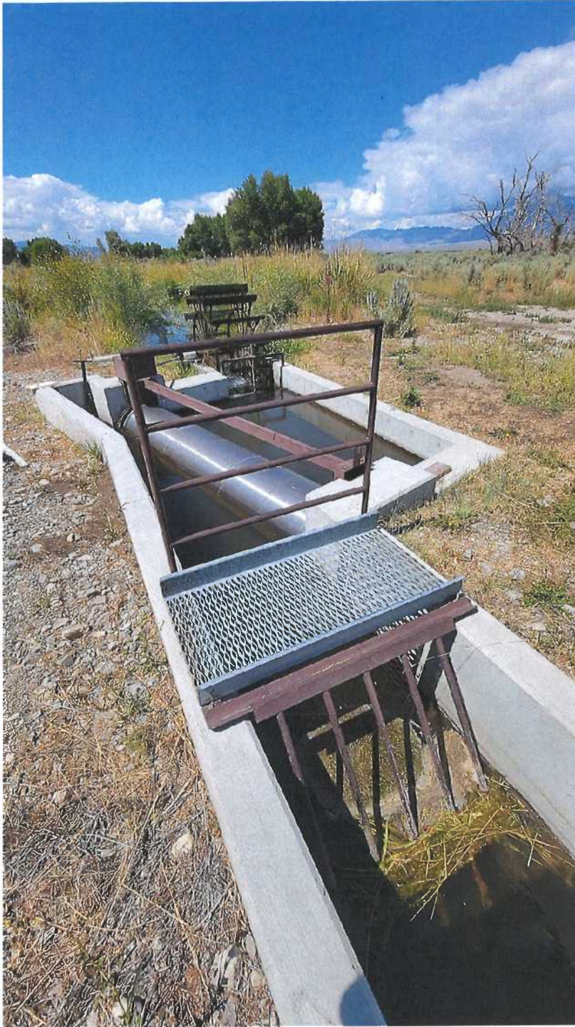
Photo 3: Approach to fish screen and bypass structure. Fish bypass pipe is at top left of the photo.
