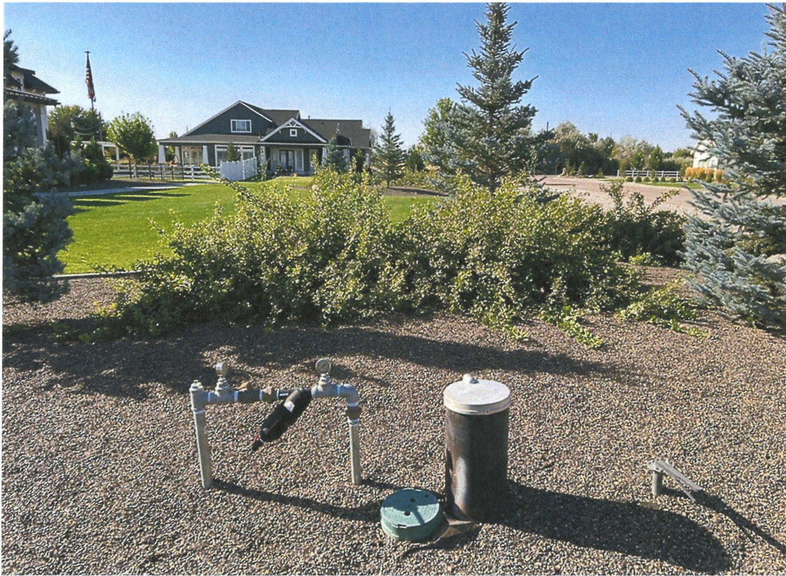
Figure 3 Photo facing south, featuring the well head and pressure gage for this water delivery system.
