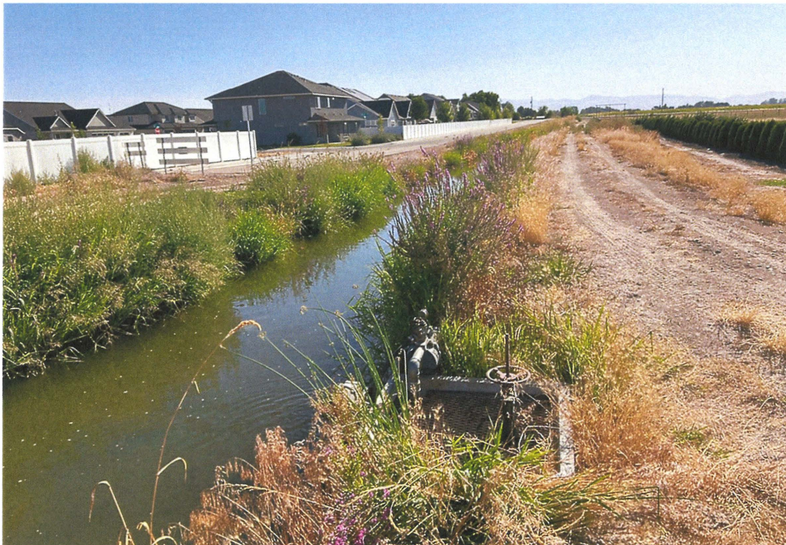
Figure 9 Headgate diversion associated with irrigation from Middleton Mill Irrigation Company. Headgate is located on north end of subdivision.
