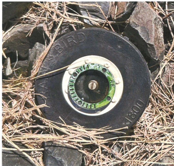
Figure 11 Rain Bird 1800 sprinkler head with H series nozzle.
