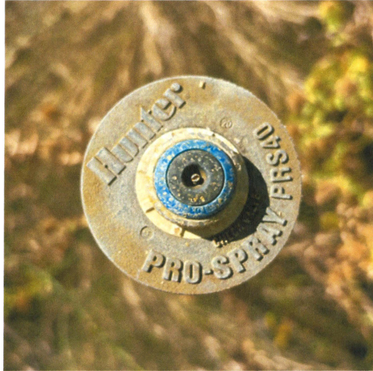
Figure 7 Hunter Pro-Spray PRS40 sprinkler head used to irrigate the perimeter of the owner's property. Another type of sprinkler is also used to irrigate the places of use.
