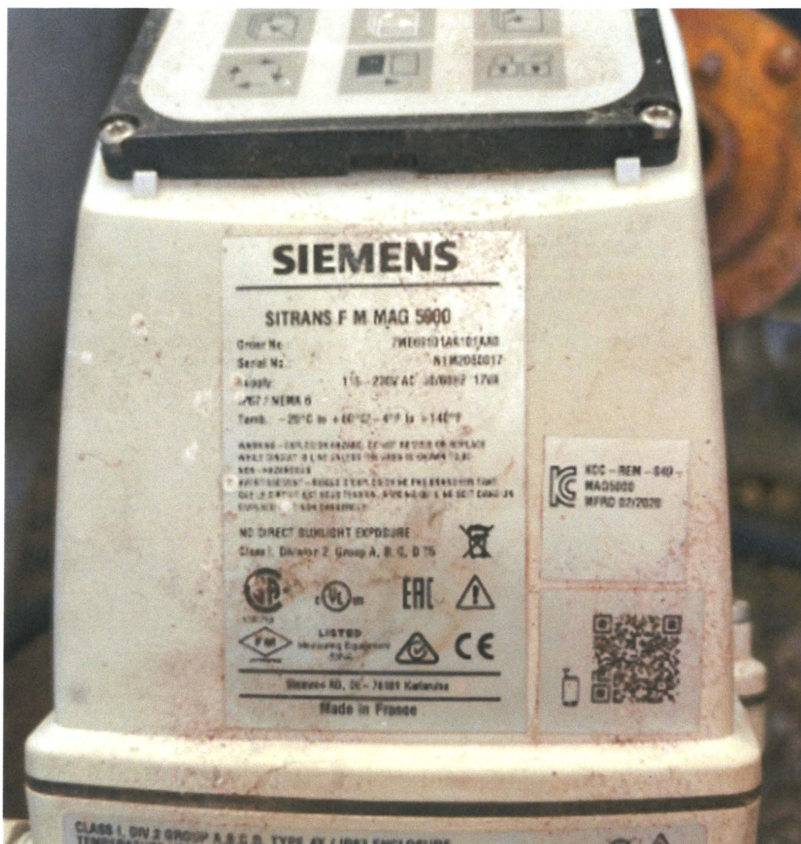
Figure 9 Specifications label for Siemens Sitrans Mag 5000 electromagnetic flow meter.
