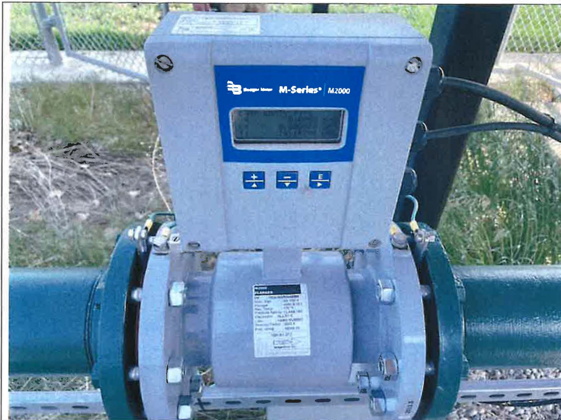
4" Electromagnetic Flow Meter
