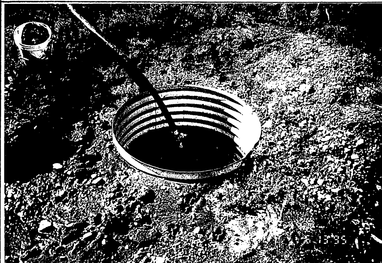
PIPE MANIFOLD NEAR WELL
