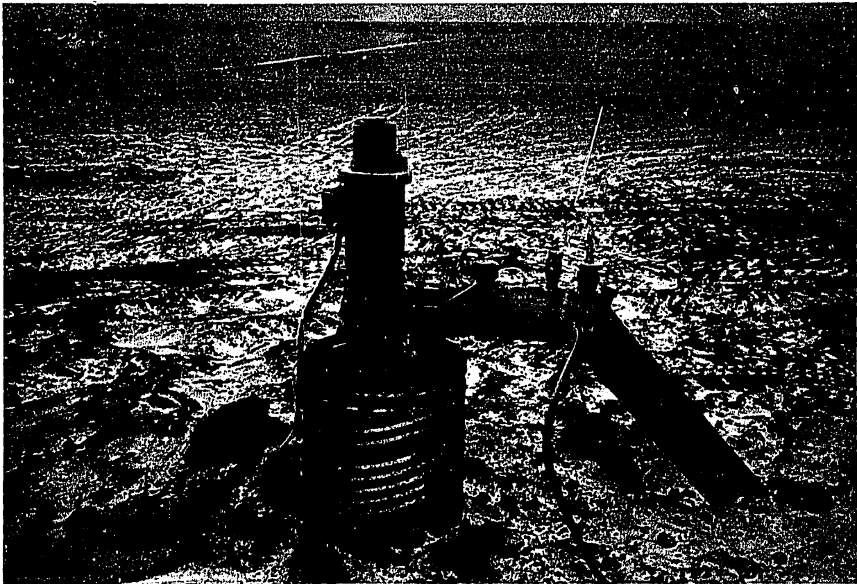
Motor & pump at top edge of Pond
