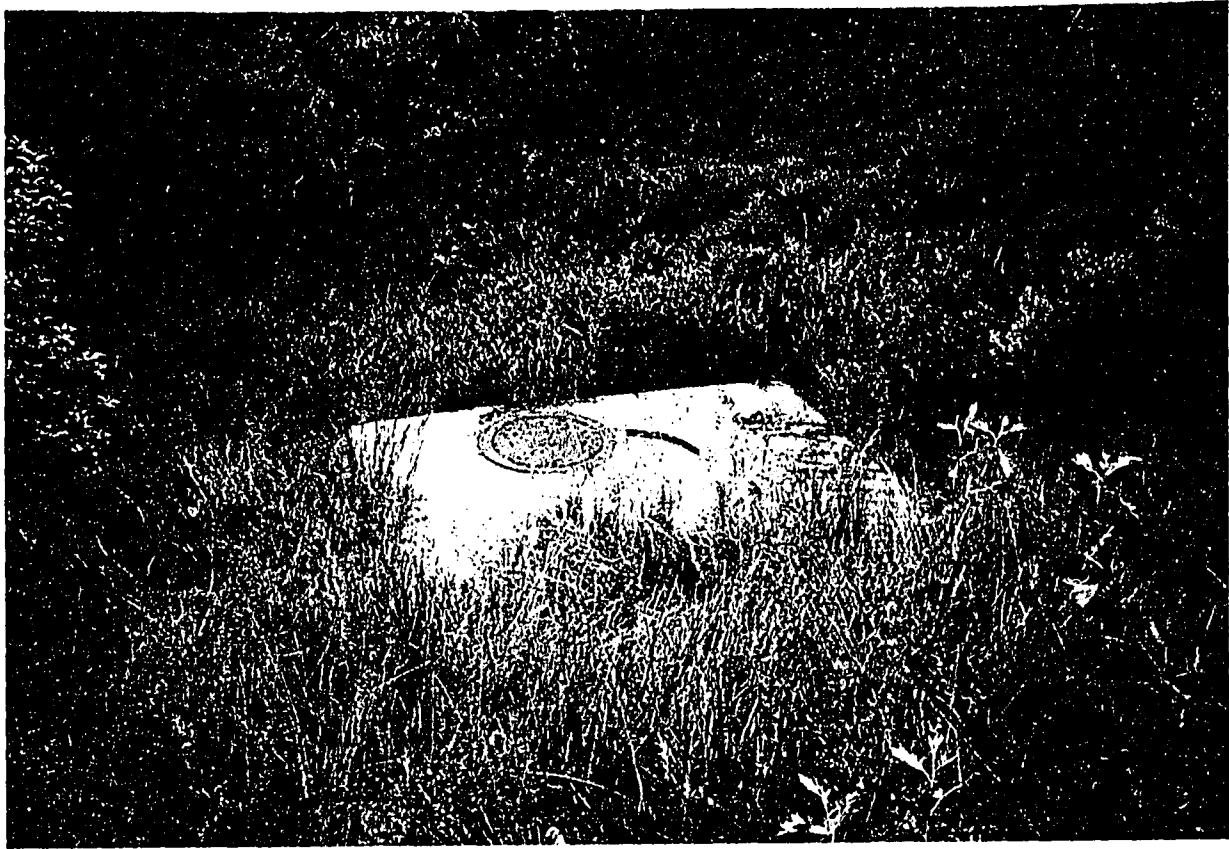
13-07544 Concrete Collection box. Springs are piped in from Right and South Top Looking South
