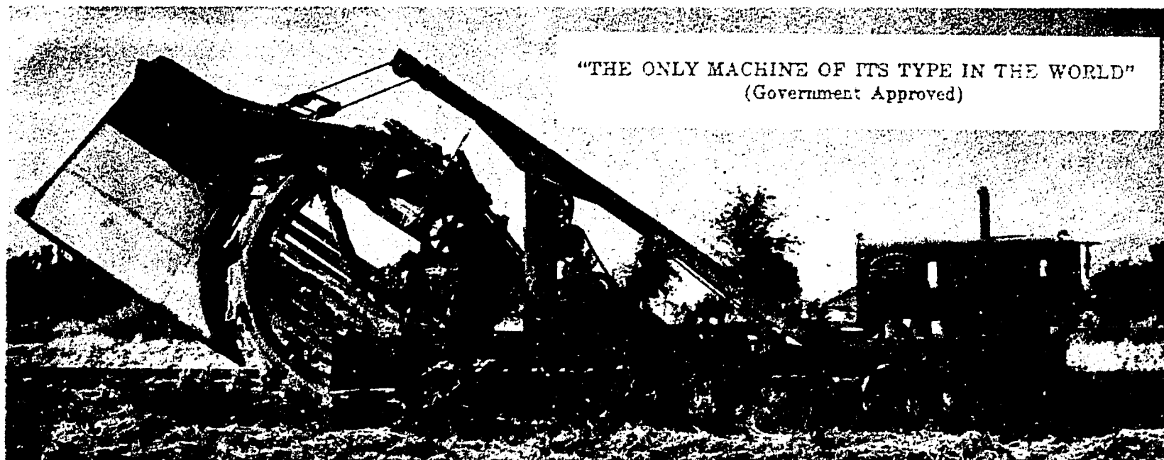
Top—Machine to dig trench, lay pipe and apply gravel filter in one operation is invention of the late Sumner G. Margetts. Device is manufactured at Layton shop.
