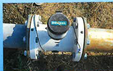
Siemens Sitrans F M Mag 8000, battery operated, external power not needed , internally grounded. Protect meter readout from weather.
