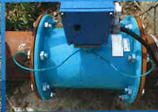
Siemens Sitrans F M Mag 8000, battery operated, external power not needed , internally grounded. Protect meter readout from weather.
