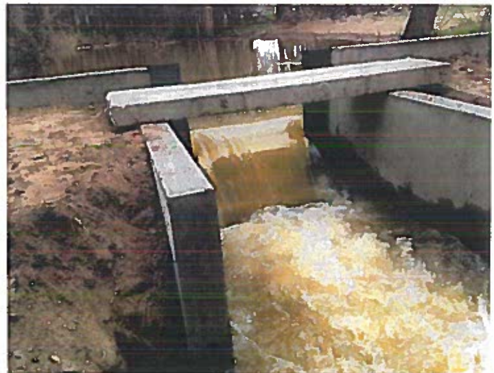
4 – foot rectangular contracted weir with staff gage (on bulkhead) and stilling well (for monitor equipment) placed in ditch above reservoir, near park office.
