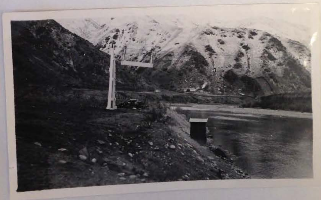
Gaging Station on Boise River below Moore Creek, looking downstream.
