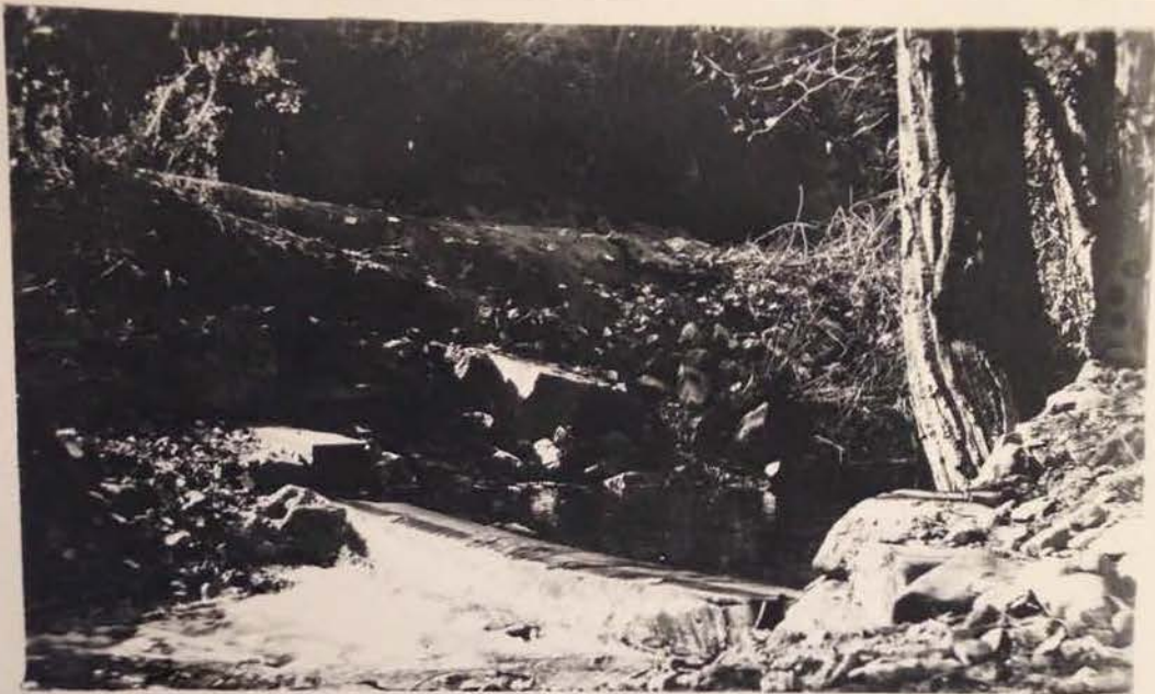
Artificial control on Cottonwood Creek during low water.
