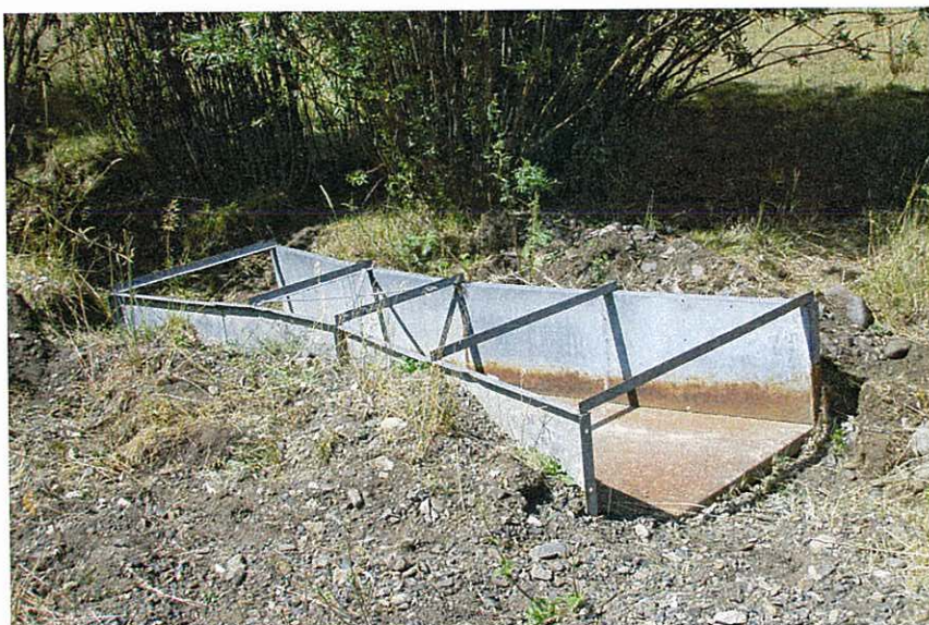
ABOVE: View on 9/6/2007 showing the control works (metal slide gate structure) on the Clark middle diversion ditch. This view location is about 200 feet downstream of the head of the “new” Clark middle diversion ditch (2 nd view on previous page). Fill material had been placed in the “old” Clark middle diversion ditch upstream of this location essentially blocking off the old ditch so that only water from the “new” diversion can reach the location shown in this view. The approximate location of the measuring device (shown in view below) is indicated. Note that during the September 2004 inspection, no control works or measuring device was present at the Clark middle diversion.
