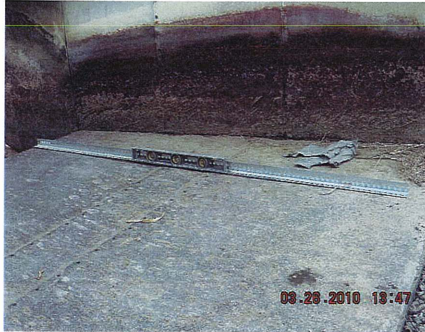
The West Side
