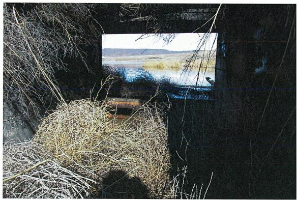
Dense tumbleweeds on the downstream side of the boards; some tumbleweeds and driftwood on the upstream slope; note that the reservoir level is below the boards at this point.
