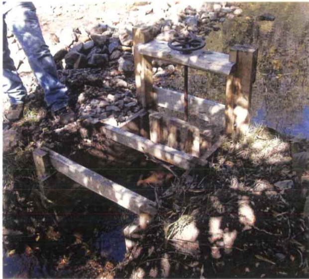
LEFT: View of wooden control works at the head of the ditch.
