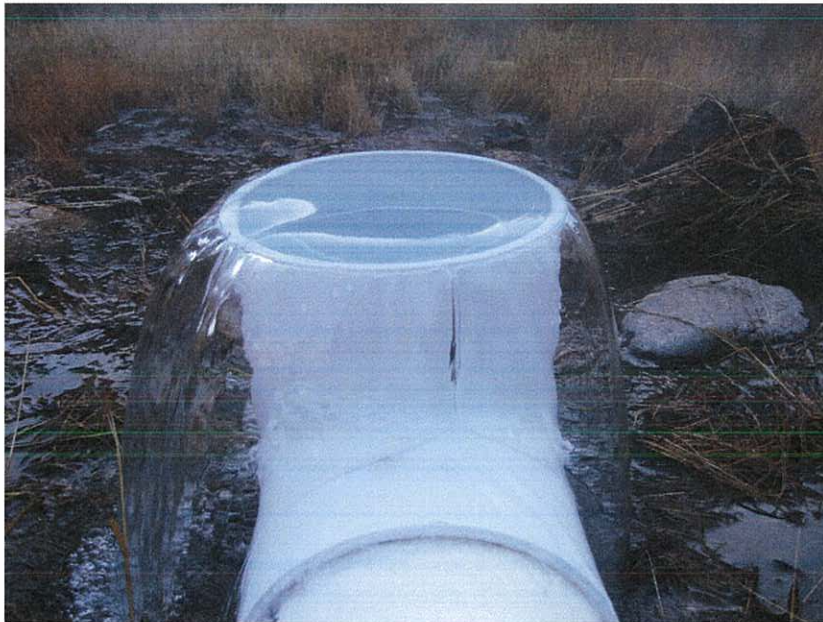
Photo 7. Pace system water issuing from discharge pipe. The elbow was installed to ensure full pipe flow so the sonic meter could be used.
