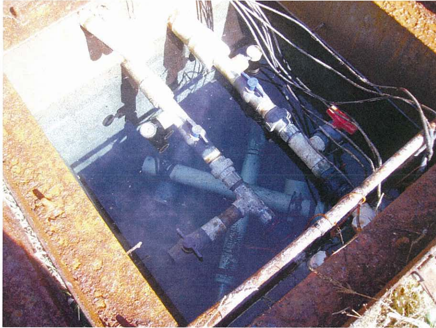
Photo 3. The Robbins sump collects water captured in perforated pipes, and submersible pumps located near the bottom deliver the water to the residence.
