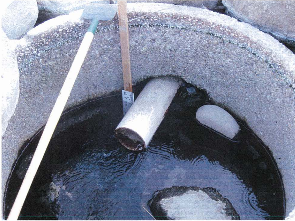
Photo 1. Pace collection system (standpipe) at “low” water level operational condition. The PVC pipe conveys the captured water to the Pace Community water users.
