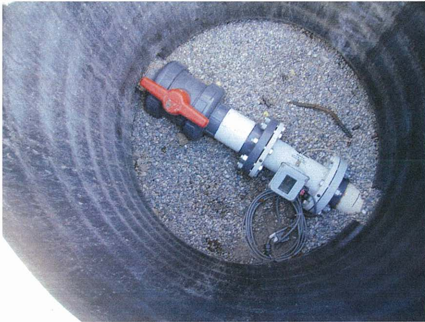
Photo 8. Robbins system magnetic flow meter. IDWR staff took hourly readings from this meter to track Robbins pumping rates.
