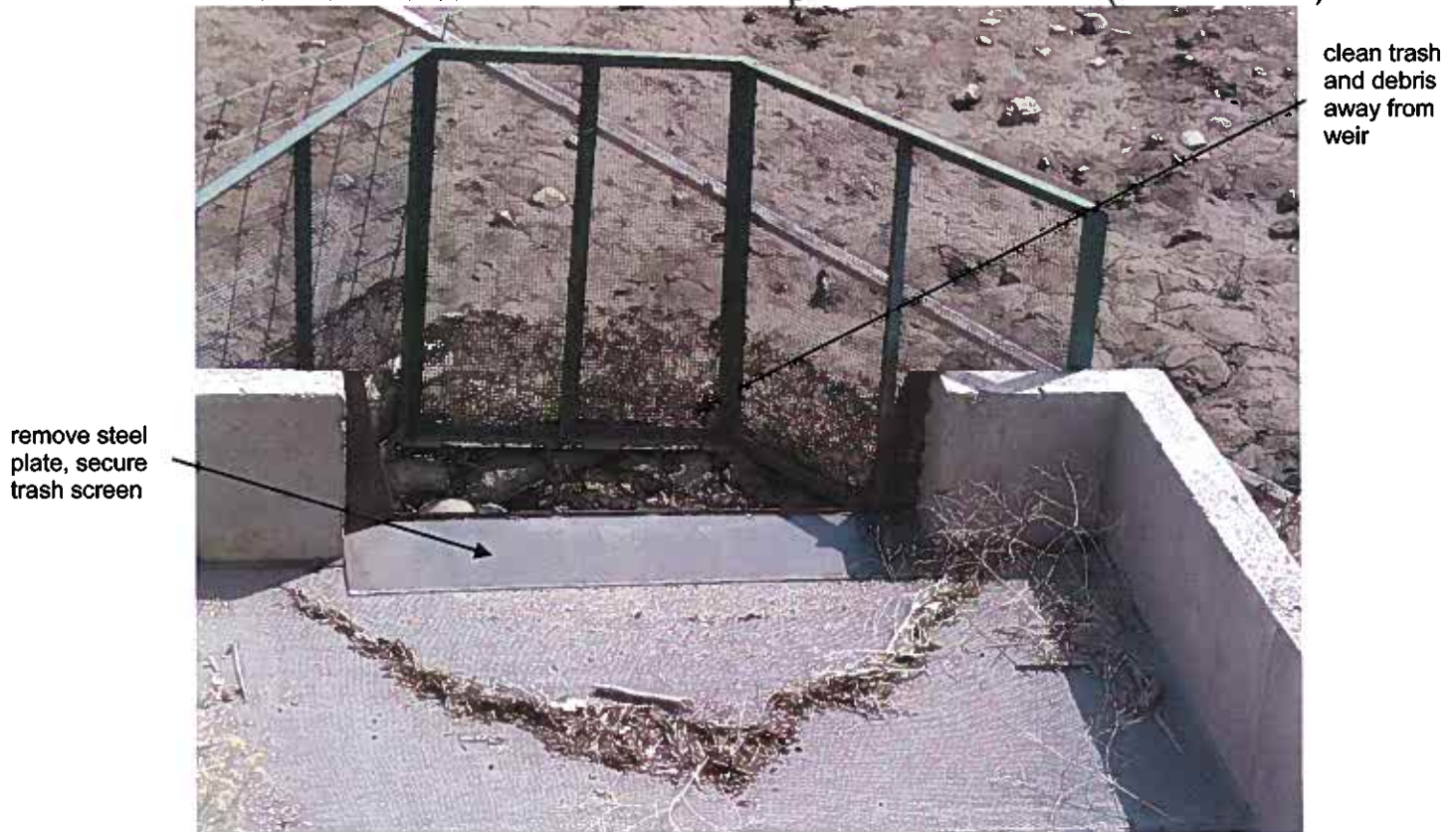
South Recharge Site weir – modification diagram
