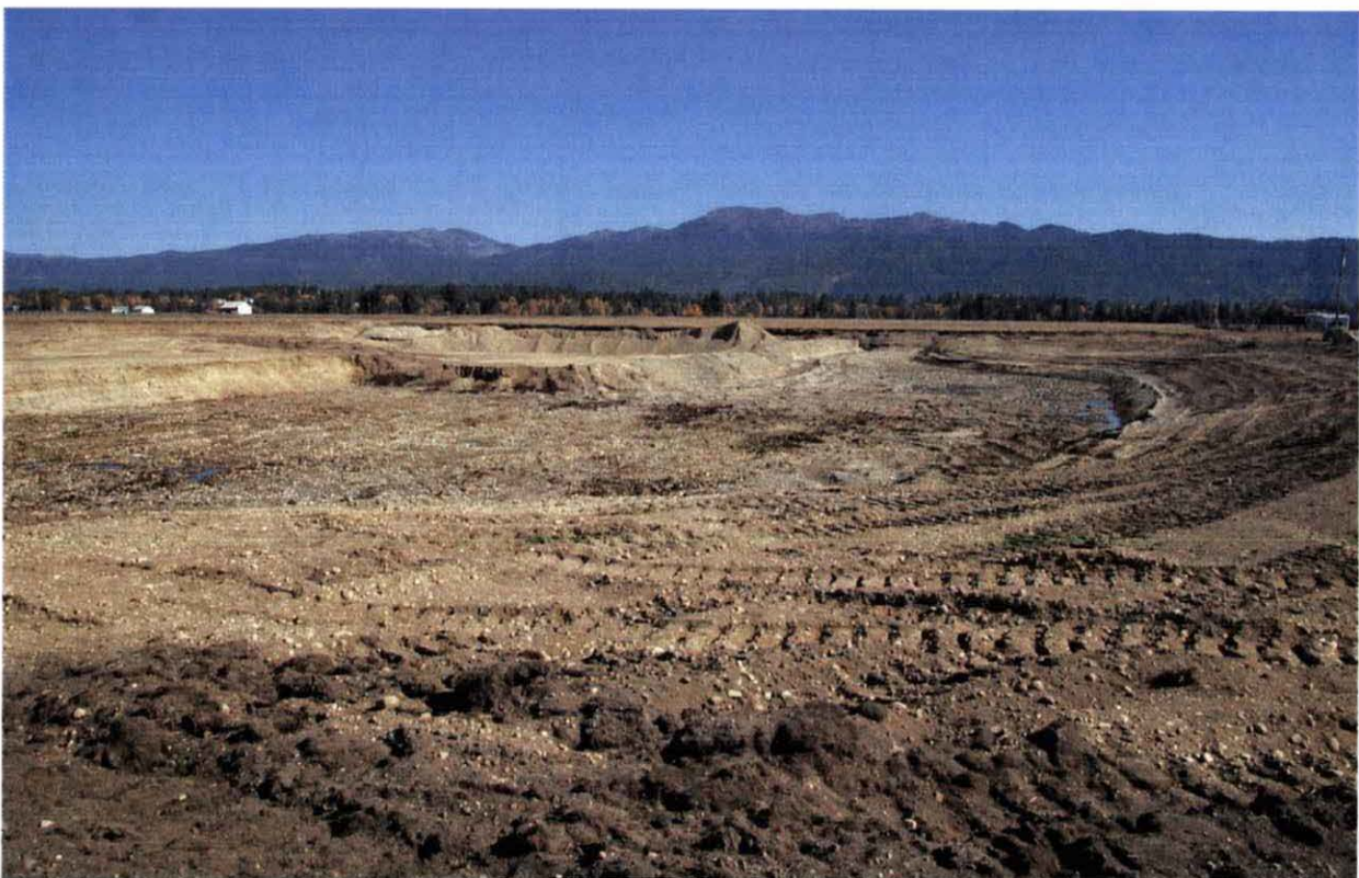
Photo #2: South ½ of the pit, some standing water along the edges, cobble rock along bottom.
