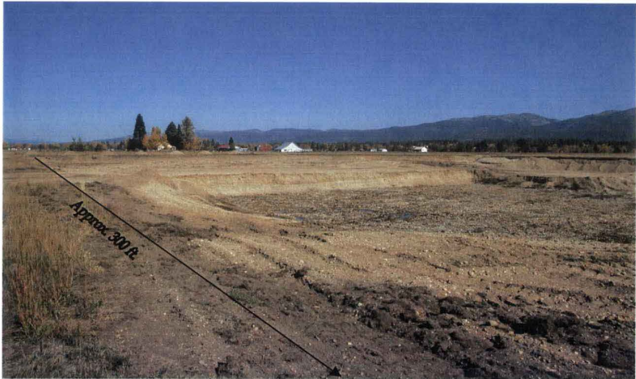
Photo #1: Pit from the southwest corner, The southwest ¼ is approx. 5 ft deep.
