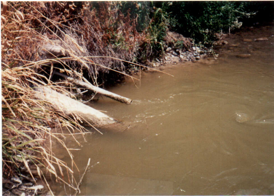
#1 Diversion pipe from Snake River.
