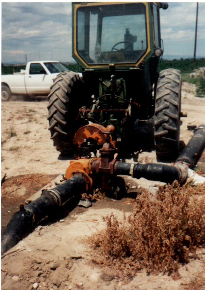
#2 Power source and pump.
