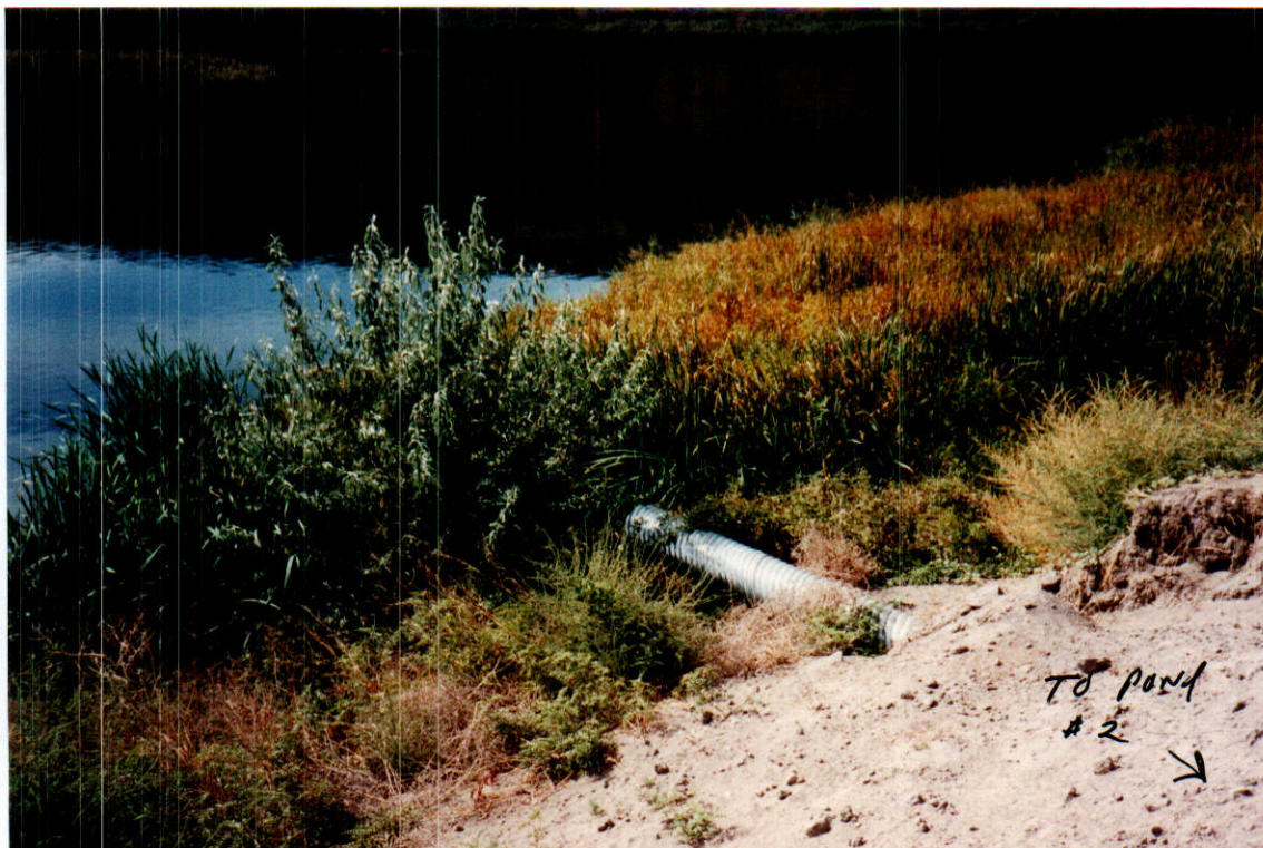
PHOTO FOUR- Return flow to river upstream from 12" culvert. Located in SWNWNG Lot 2. Overflow from Pond #2.
