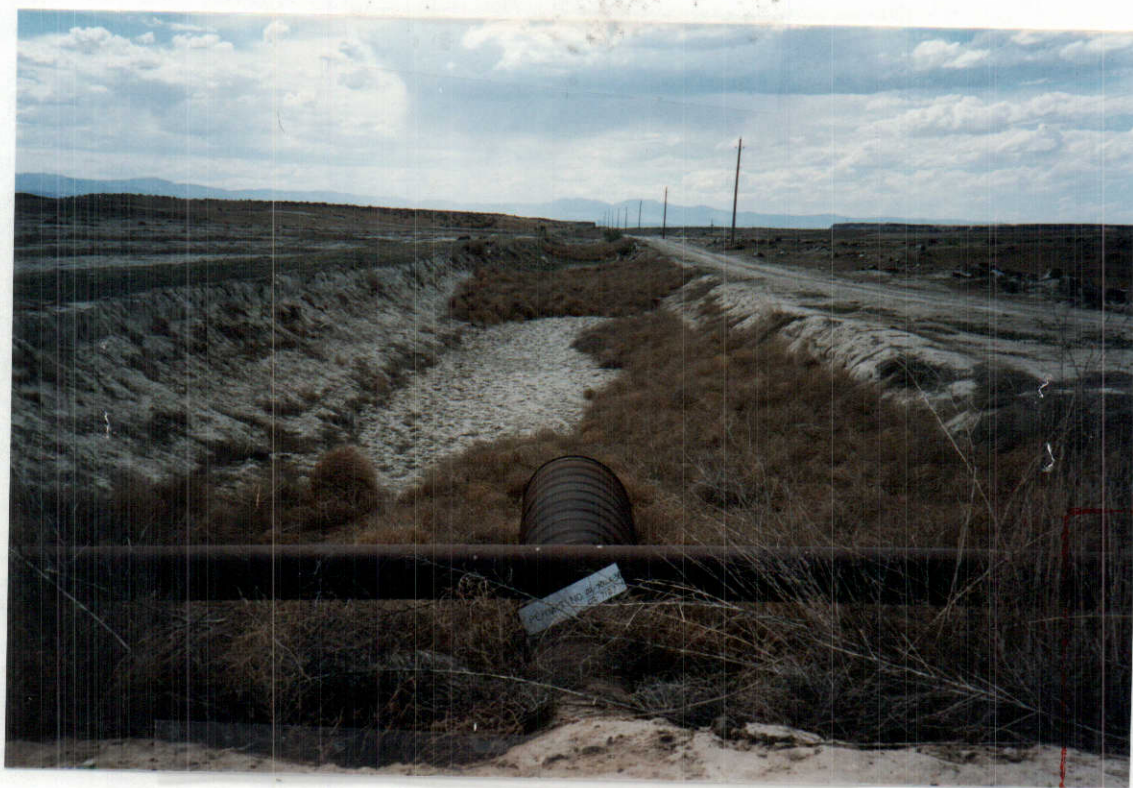
END of ENLARGED DITCH Looking West
